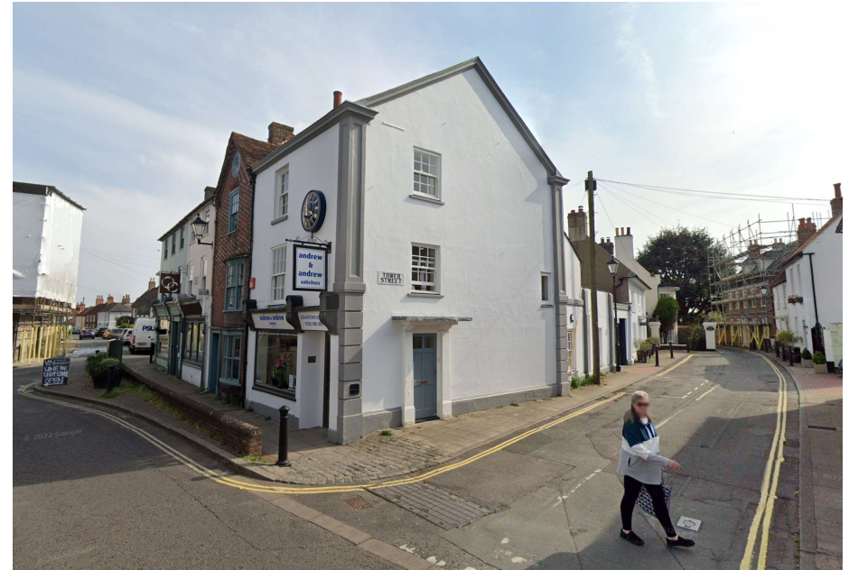
Existing Building fronting High Street and Tower Street
