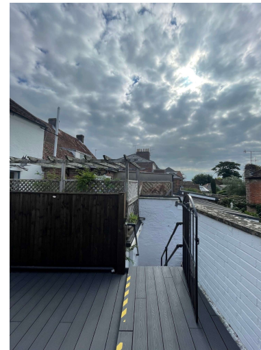
View from Existing Terrace – Looking S.E
