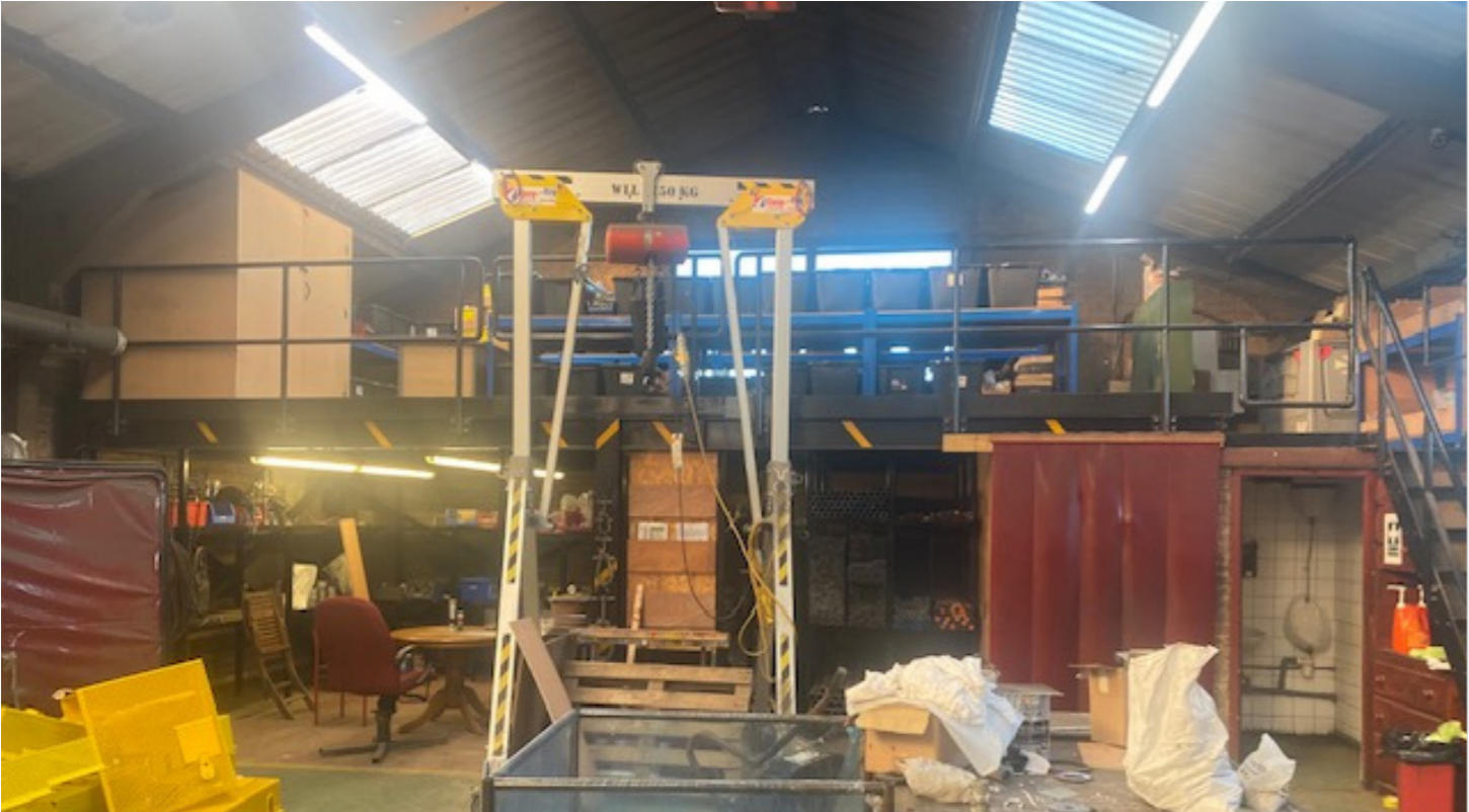
View of the mezzanine within the warehouse/workshop
