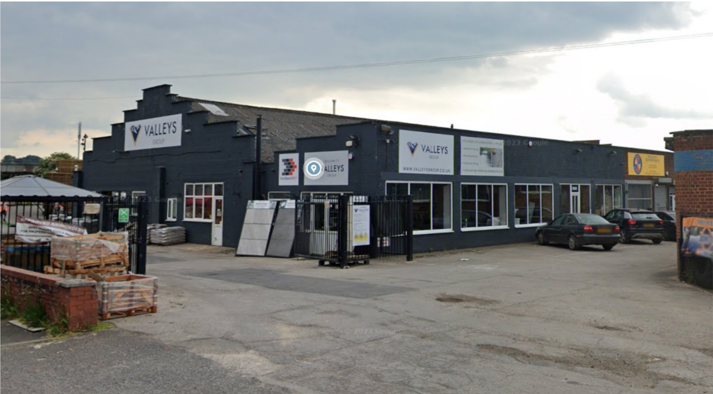
3. Existing large brick existing building South, East of the proposed site
