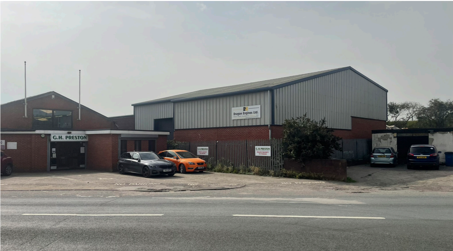
1. Existing neighbouring property, West of the proposed site
