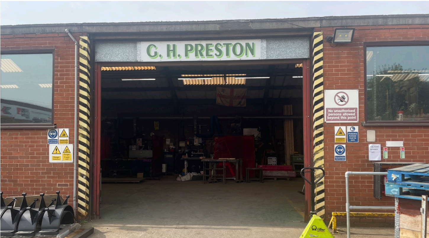
Existing warehouse/workshop entrance
