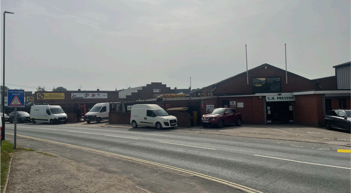
Existing building, view looking East
