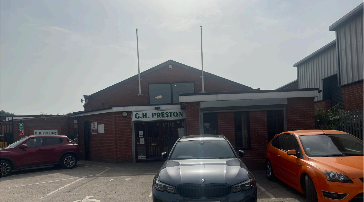
Existing building, view looking South
