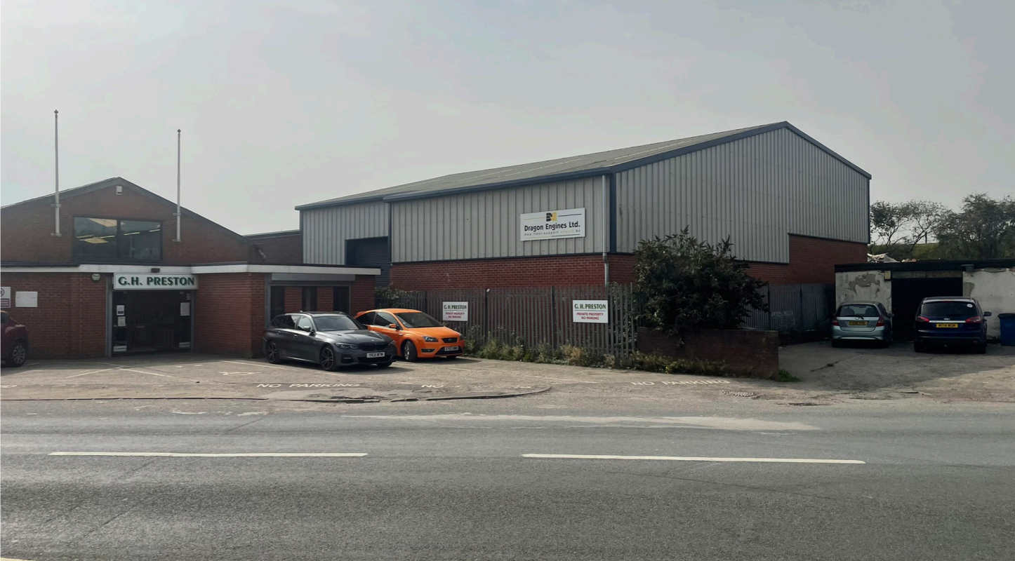
Existing building, view looking West
