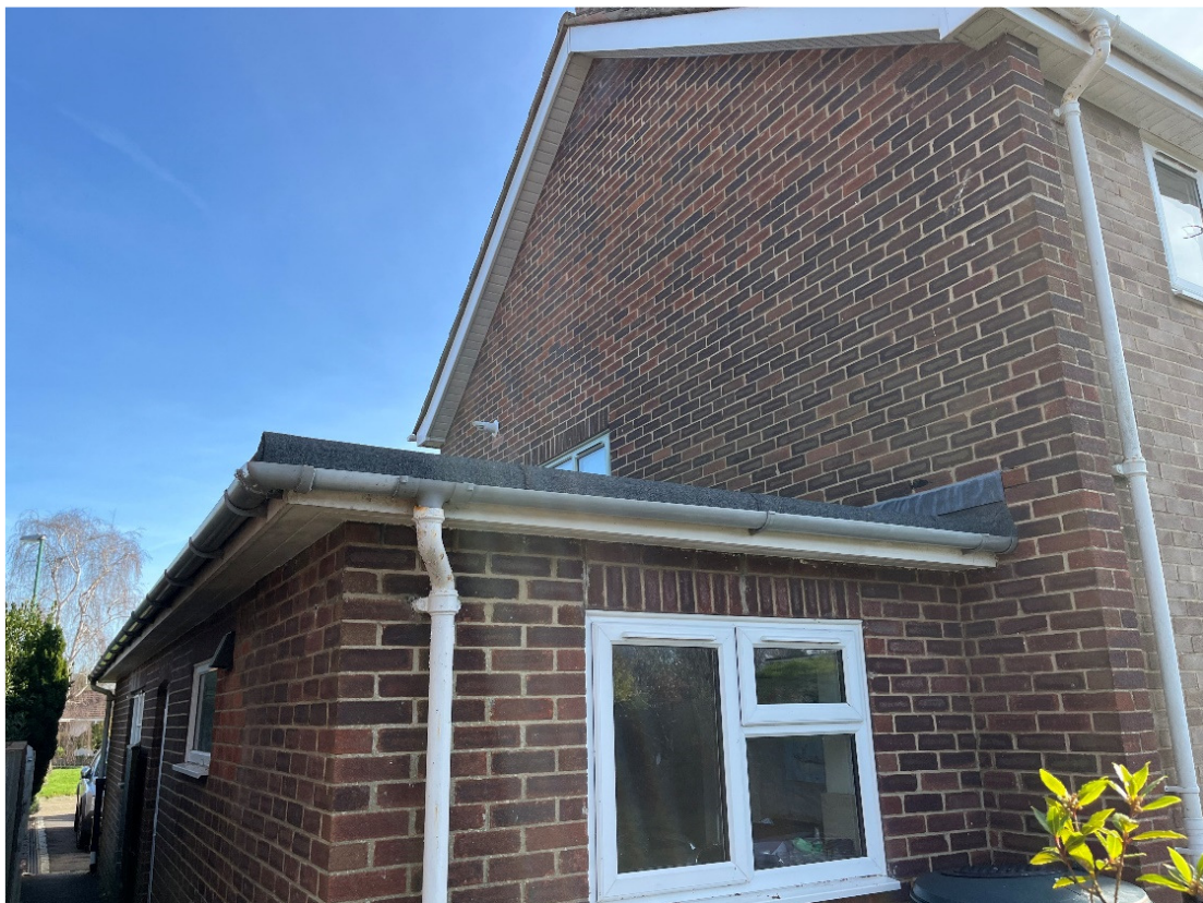
Figure 4. Garage and house northern elevations looking east.
