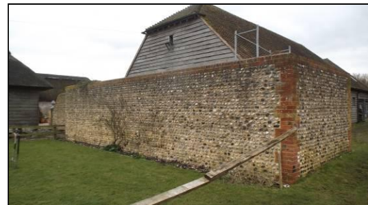
The north end of the farmyard wall, from the north-east.
