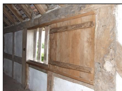
A typical window opening and a sliding shutter.
