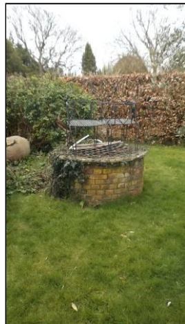
The well head, from the east.
