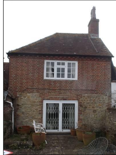
The west elevation of the west extension.
