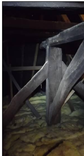
Truss 1, from the south-east (right) and from the north-east (far right).
