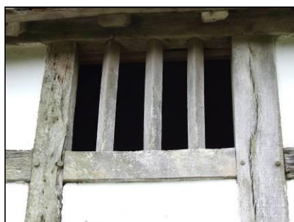
A typical window opening and a sliding shutter.
