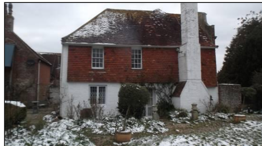
South Mundham House, from south.
