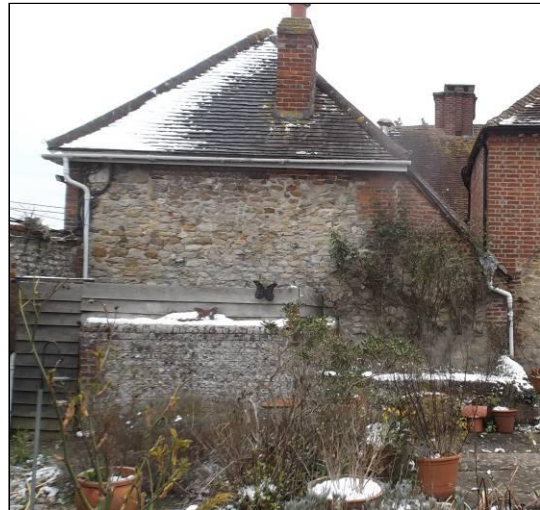
The west wall of the north range.
