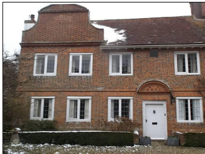
The southern part of the east elevation.
