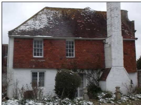
The south wall of the south range.
