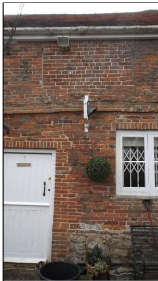
The blocked window opening over the stable door.
