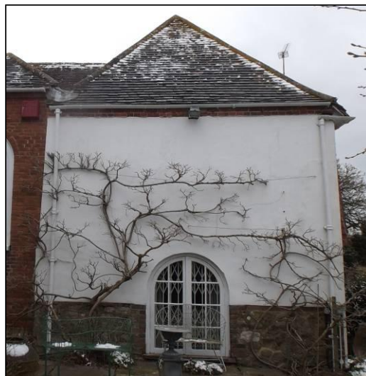
The west wall of the south range.
