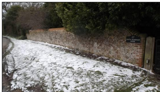
The boundary wall (a-b), from the north-east.
