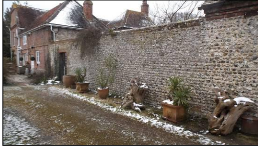
The garden wall (g-h), looking east.
