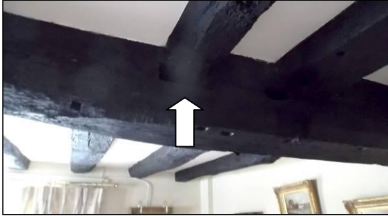
The re-used mortice (arrowed - above left) and the inserted timbers, looking east (above right).
