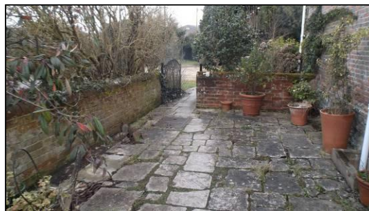
The garden wall (e-f), from the west.
