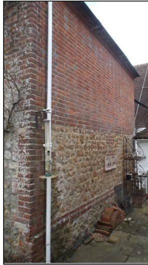
The east elevation of the west extension, from the south-east.
