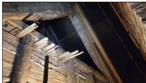
The south end of the lath-and-plaster ceiling (above) and the external face of the partition at the south end (right).
