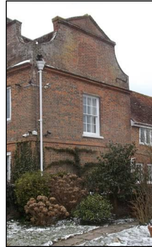
The north elevation of the east range, from the north-east.
