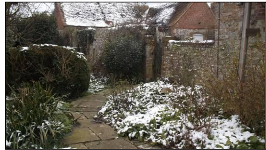
The garden wall (j-k), looking west.
