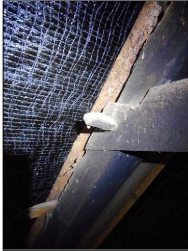
The dovetail halving joint at the south end of Truss 2 (left) and a typical joint of this type (above).
