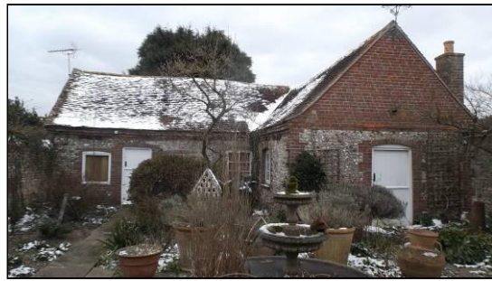
The former dairy, from the east
