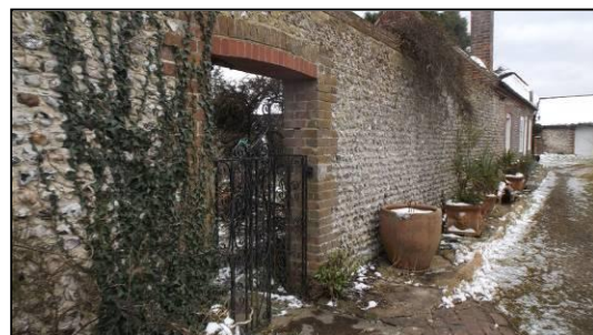
The garden wall (g-h), looking west.
