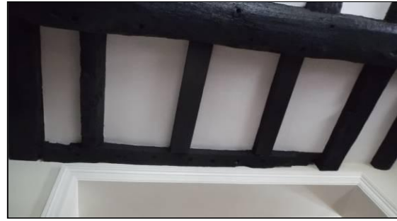
The re-used mortice (arrowed - above left) and the inserted timbers, looking east (above right).
