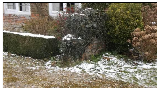
The garden wall (c), from the north-east.
