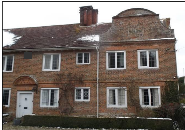
The northern part of the east elevation.
