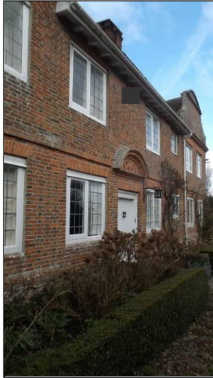
The projecting eaves on the east elevation.
