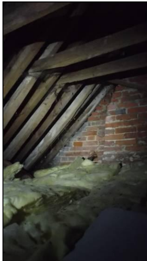
The roof of the west extension, looking south.
