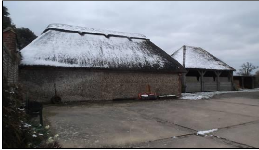
The barn, from the north-east.
