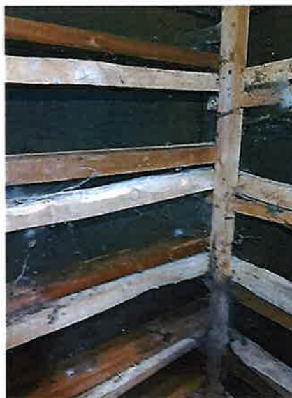
Interior of roof, SW annexe
