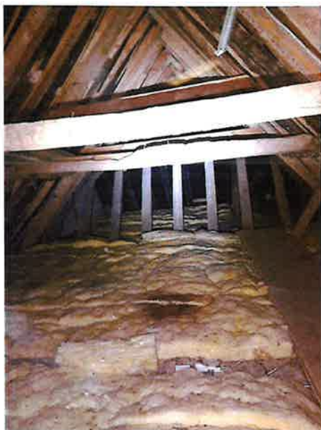
View of area of main roof void/s
