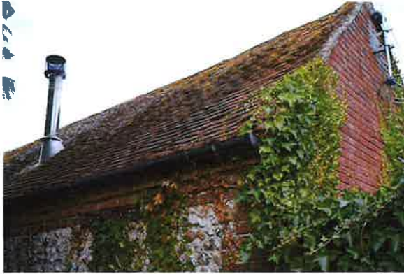
Views of exterior of outbuilding – from SE
