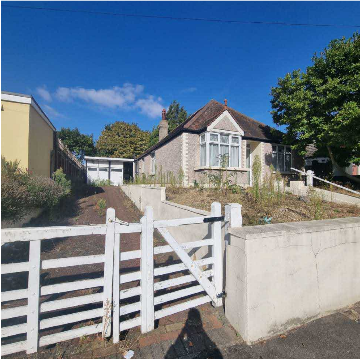
Image looking at the front of 108 Havelock Road.
