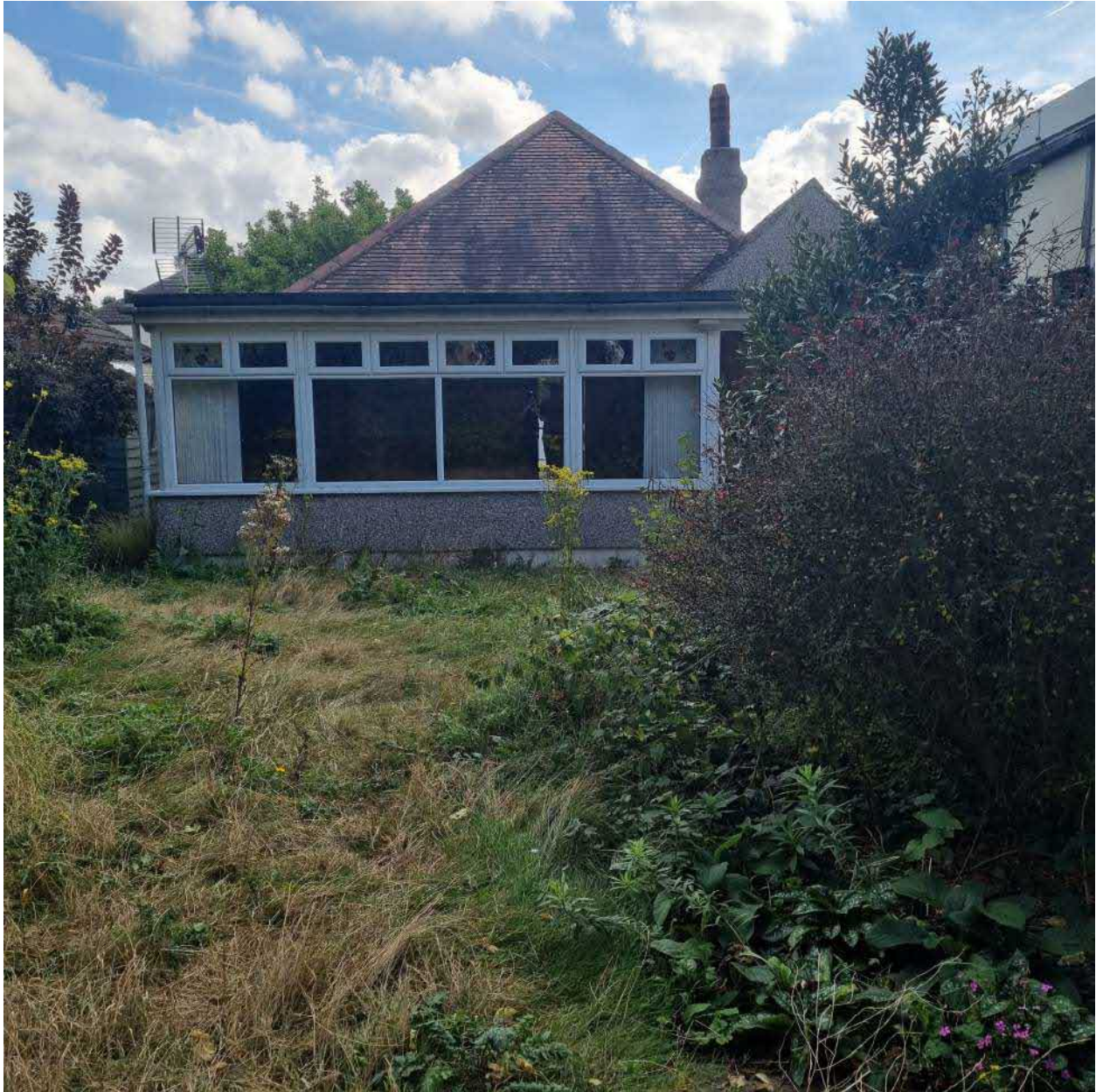
Image looking at the rear of 108 Havelock Road.
