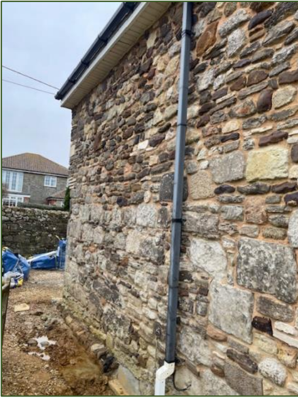
Figure 21. West facing elevation stonework; differences indicate former heightening.
