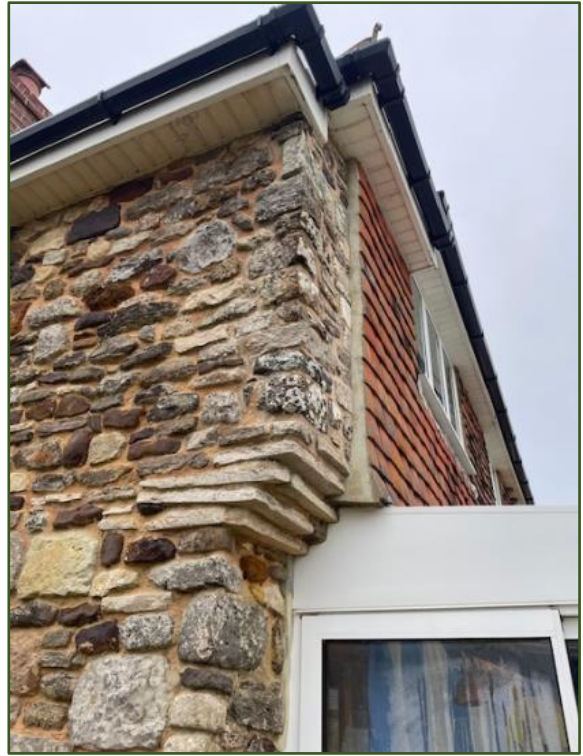
Figures 37 & 38 showing untidy arrangement of soffits, fascia boards and rainwater good due to poor design/construction of existing roof.
