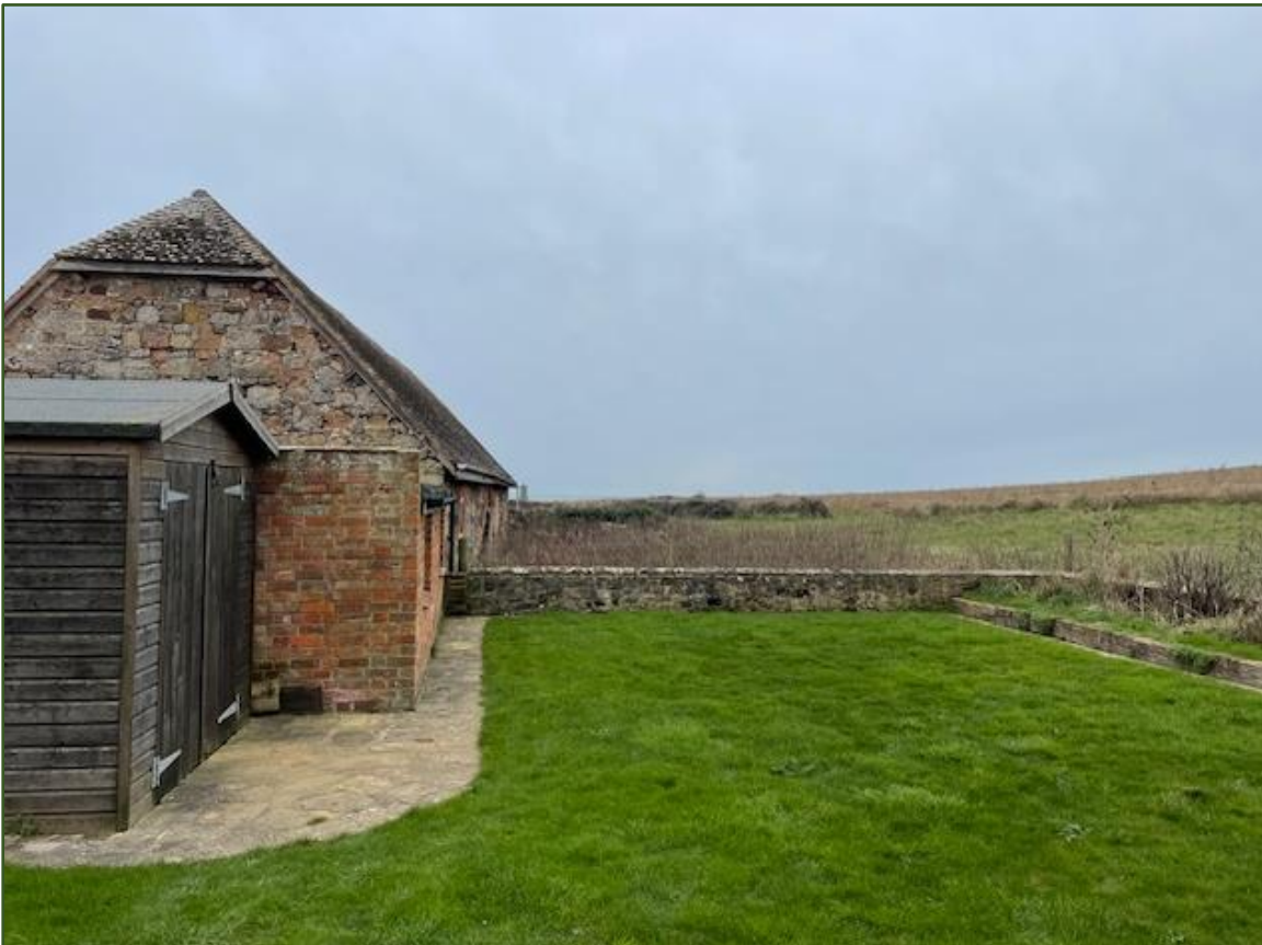
Figure 30. View from rear of The Old Brewhouse looking south.
