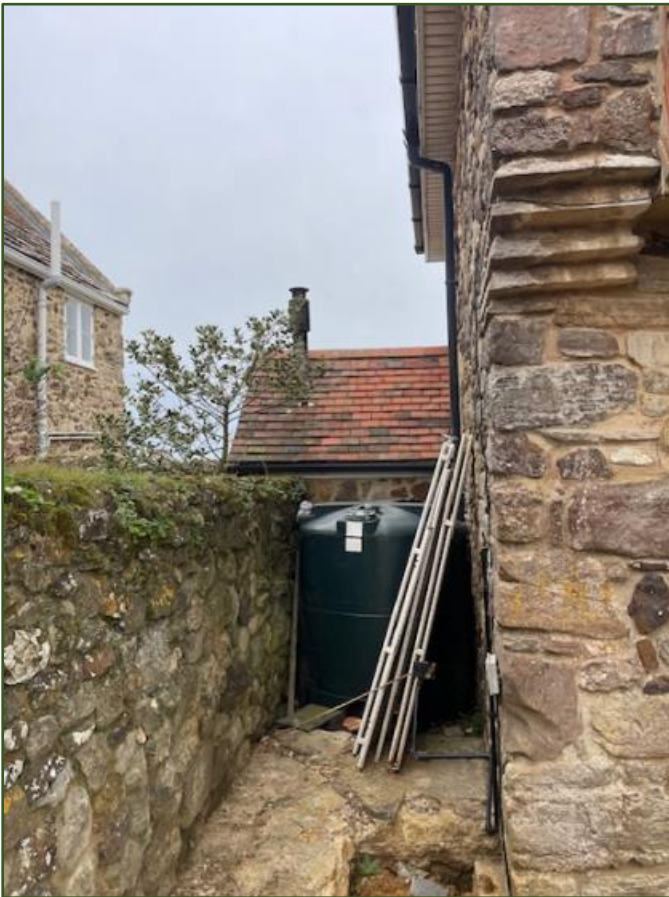
Figure 39. Oil tank to the north of porch; visible from Coastguard Lane.
