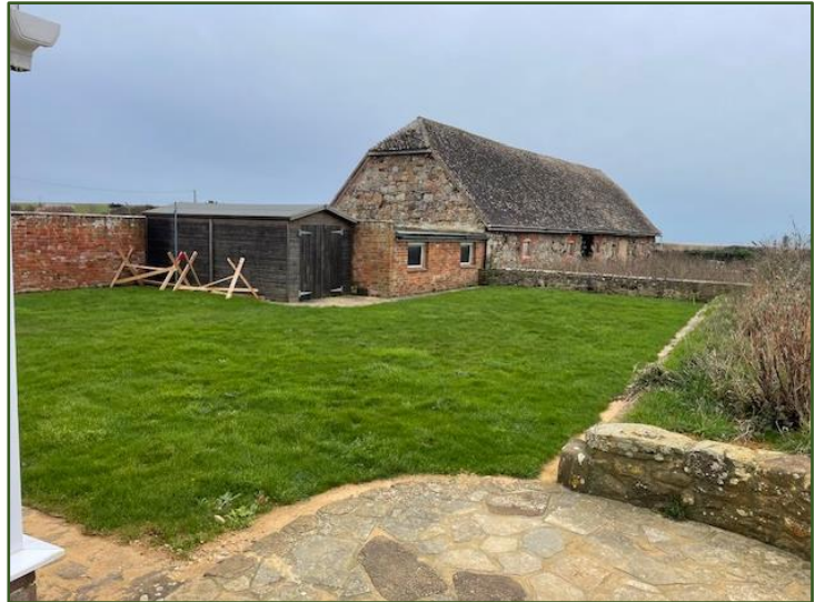
Figure 29. View to south east across garden towards old long stone barn.
