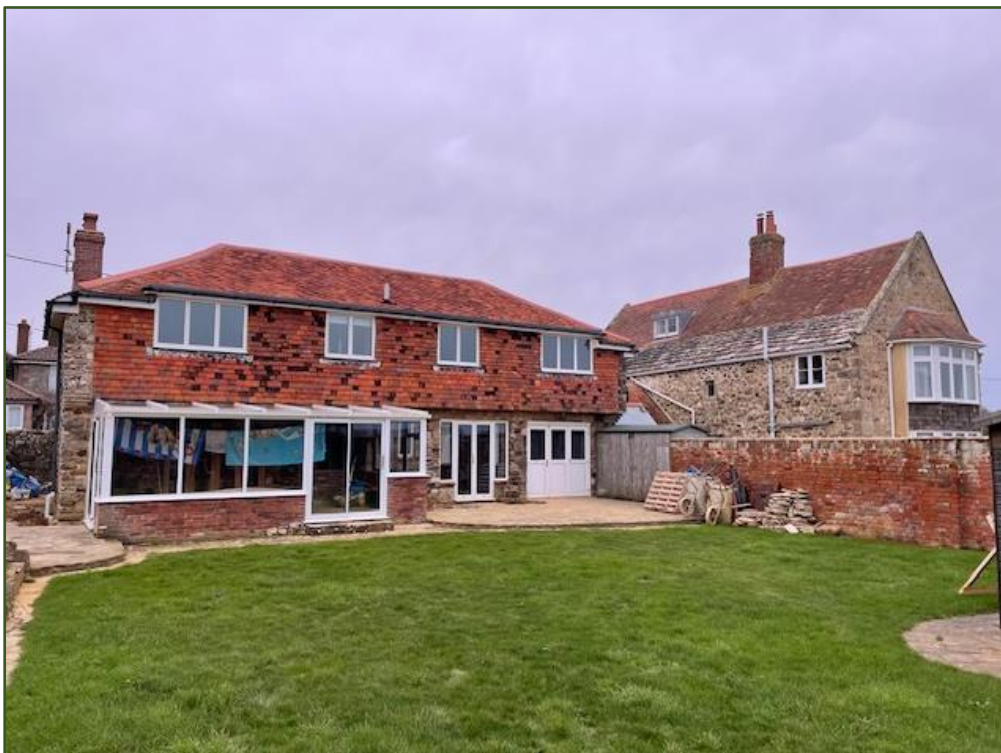
Figure 20. South facing rear elevation illustrating visual impact of white UPVC and inconsistency in fenestration. Note irregular and angular arrangement of roof/rainwater goods.
