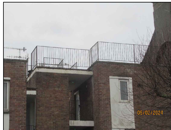
Existing roof access to north block roof
