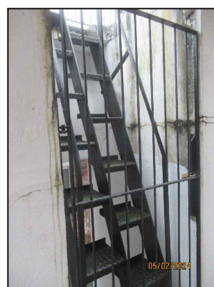
Existing Access steps onto North Roof
