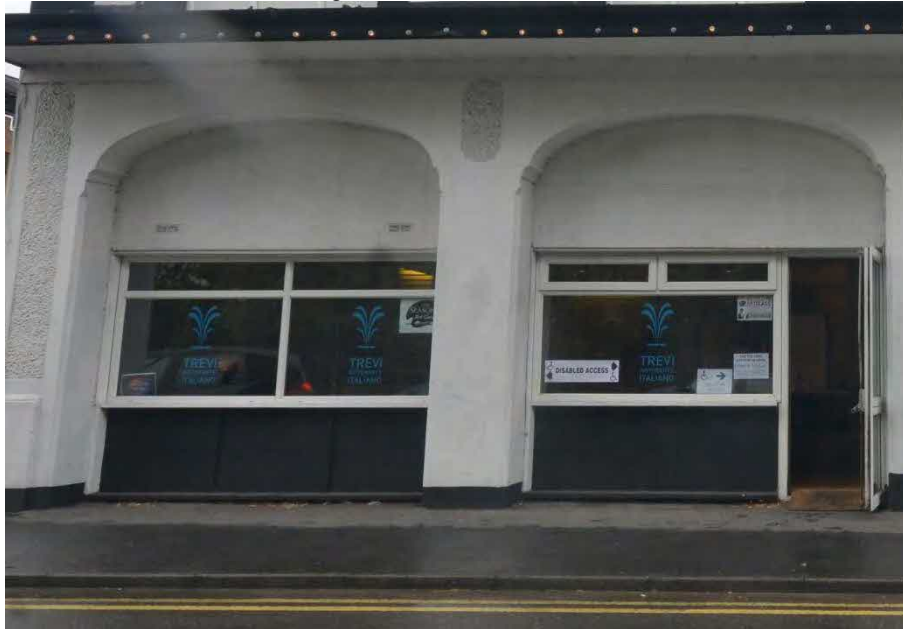
Plate 24: Unsympathetic blocking of boat house openings
