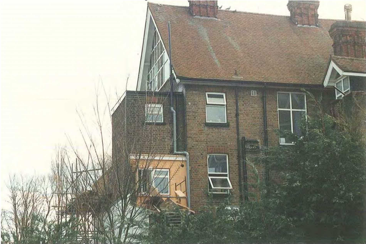
Plate 15: The northern extension, viewed from the northwest
