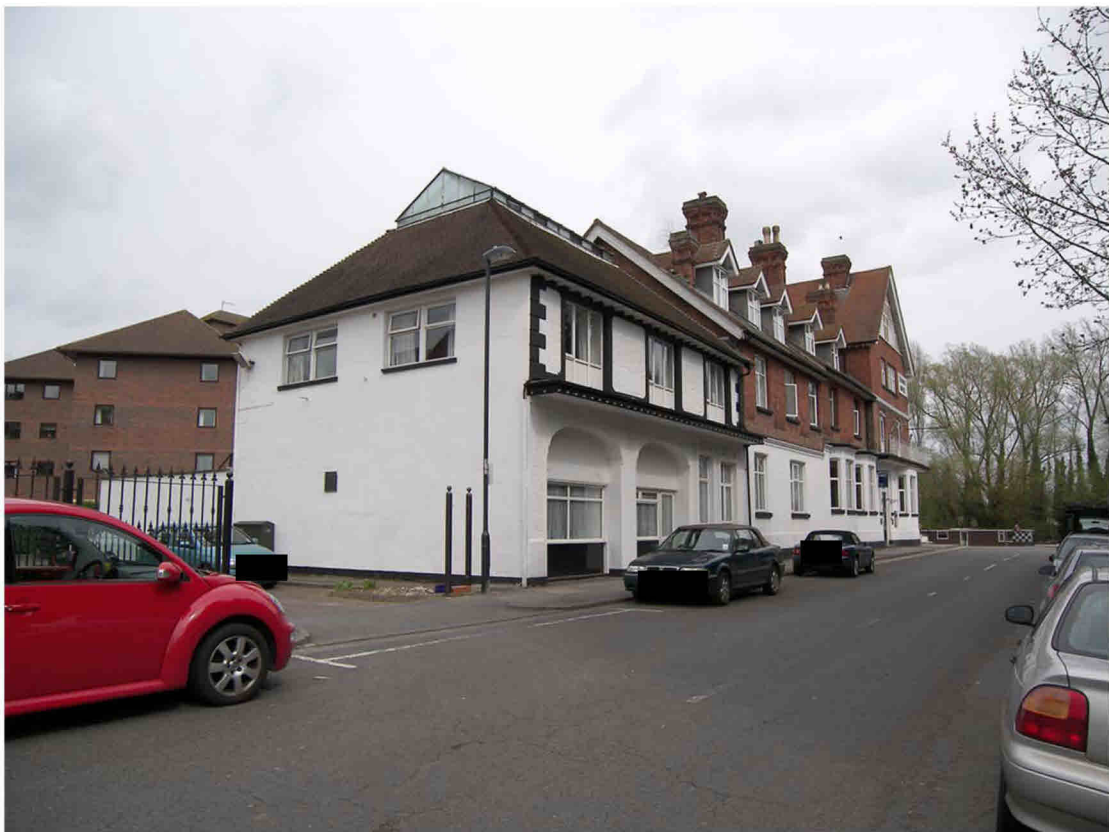
Site From West
