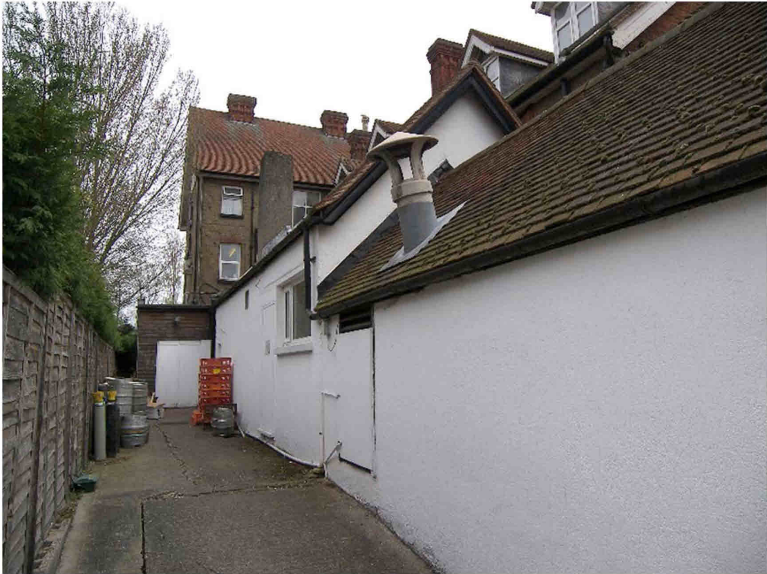
Along rear bdy of site to north sml
