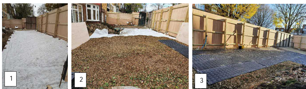
Images above from a site managed by Usherwood Arboriculture and showing the three stages of ground protection installation.
