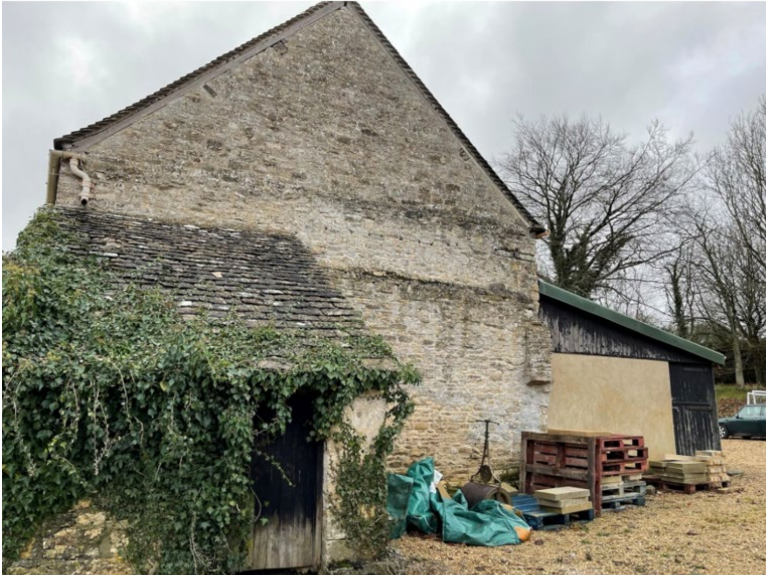
Plate 10: Listed barn, north-east flank elevation.
