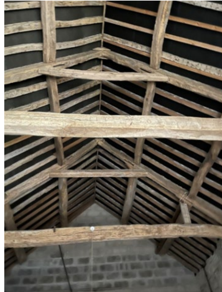
Plate 14: Detail of roof structure.
