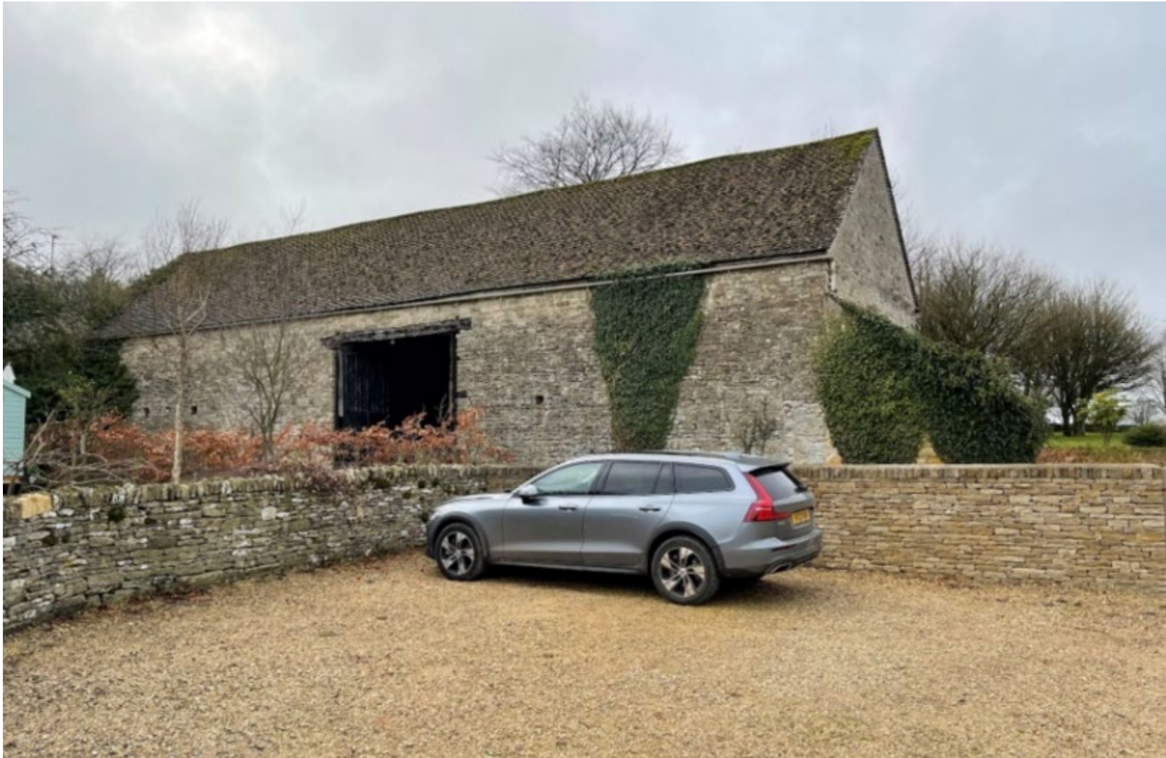
Plate 8: Listed barn, south-east elevation.
