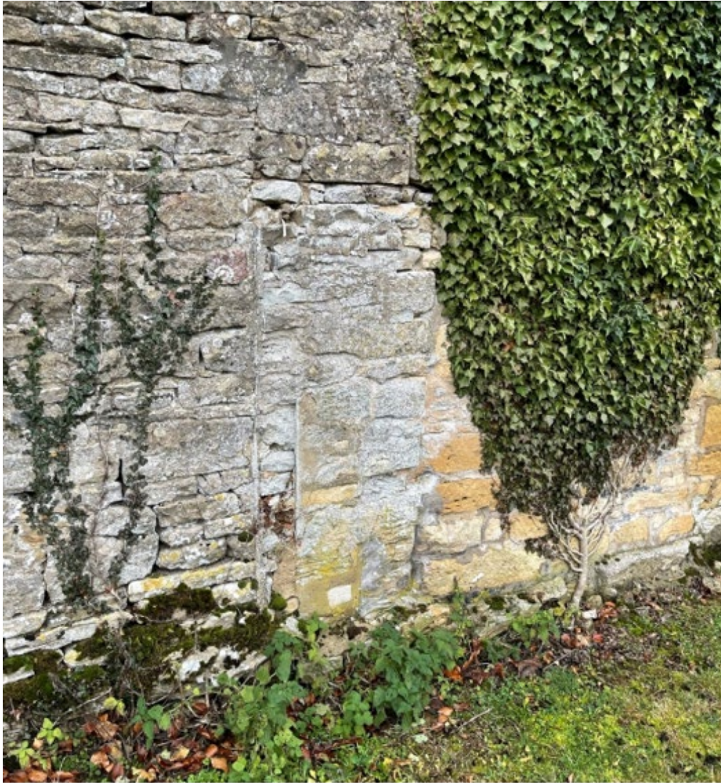
Plate 9: Listed barn, south-east elevation, detail of blocked doorway on north-east elevation.
