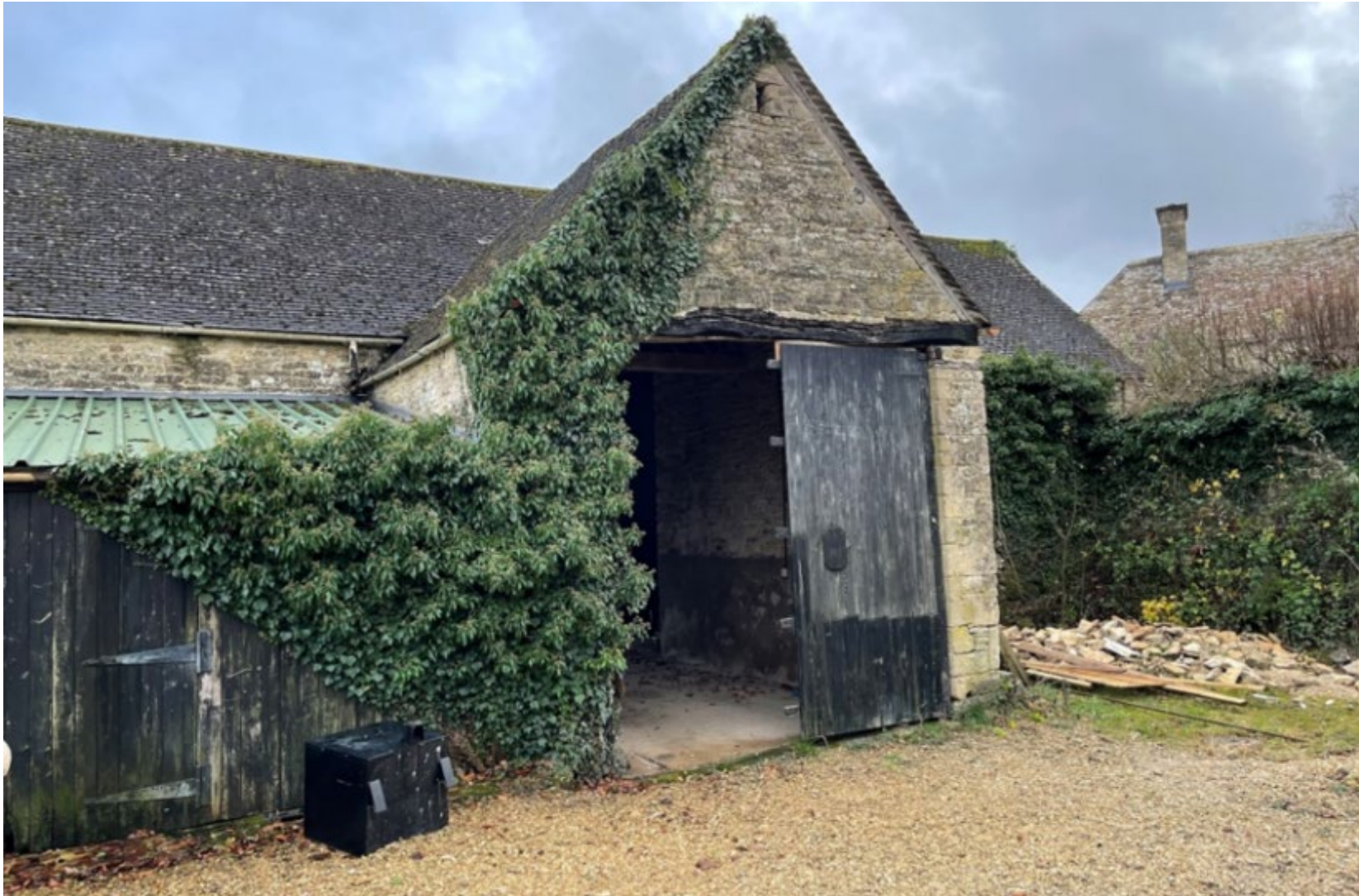
Plate 11: Listed barn, north-west elevation.
