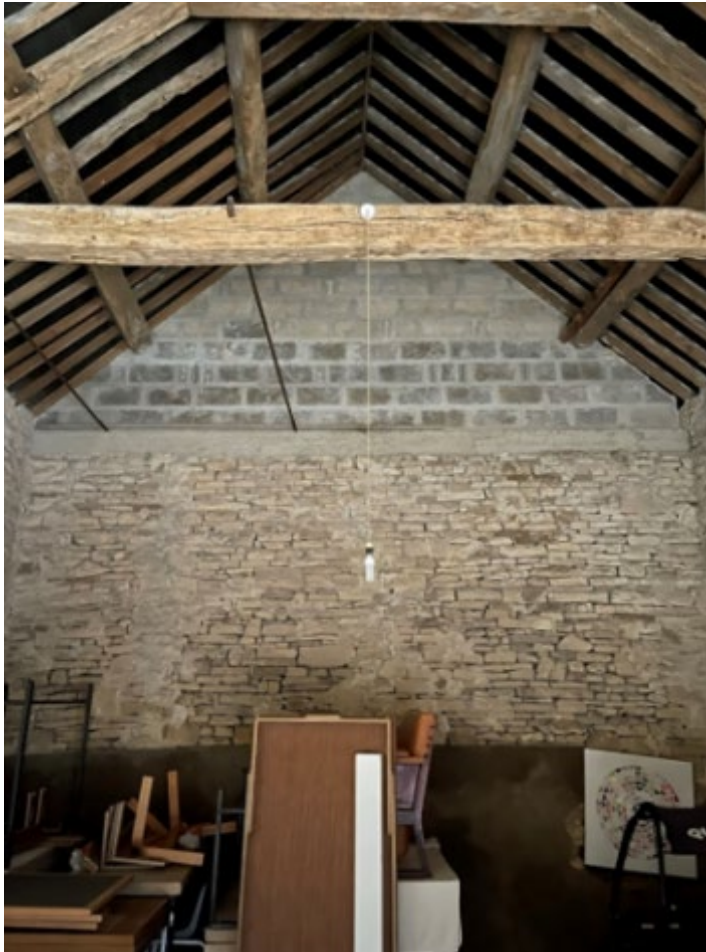
Plate 13: Interior looking towards the north-east gable wall.
