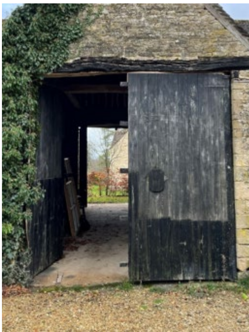
Plate 16: Detail of barn doors to north-west porch.
