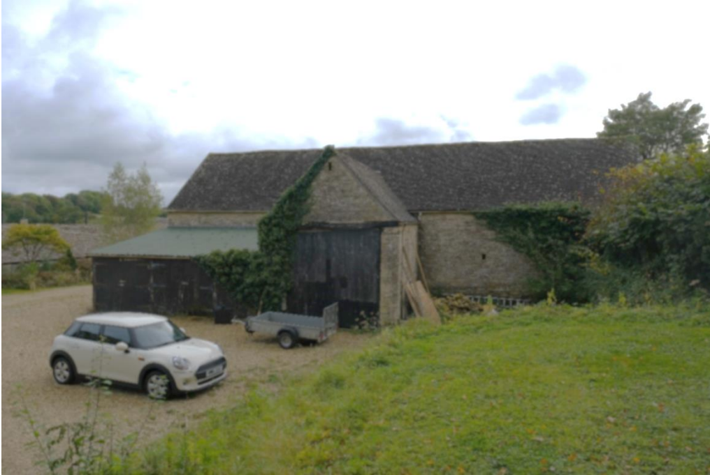
View from the rear of the barn
