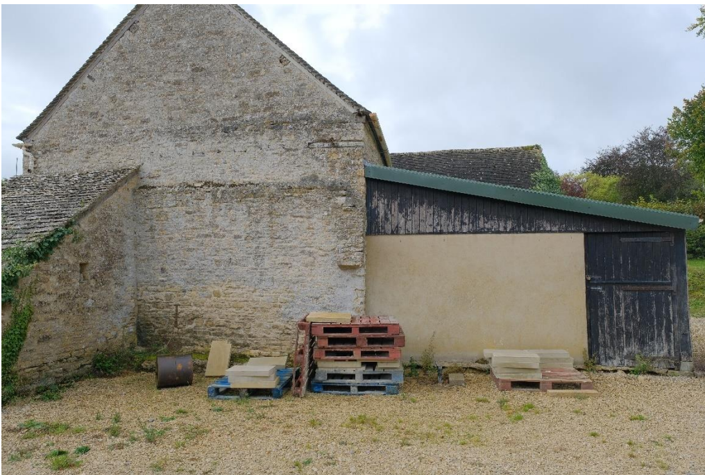
View showing modern lean to on the side of the barn
