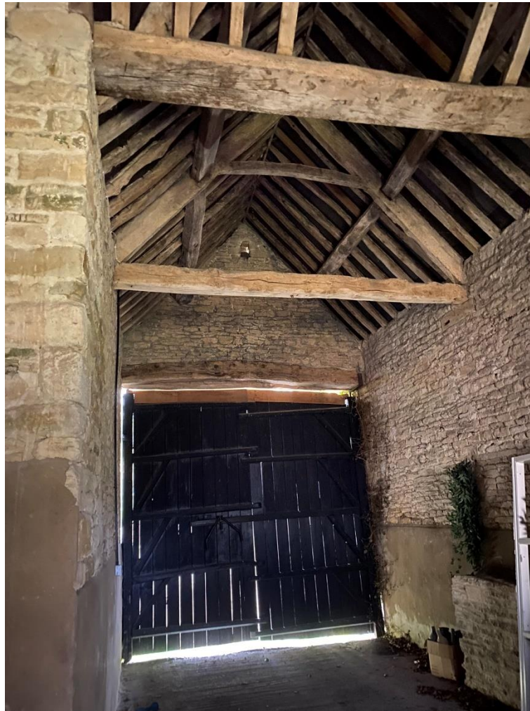
Plate 3: Internal view of barn showing doors.
