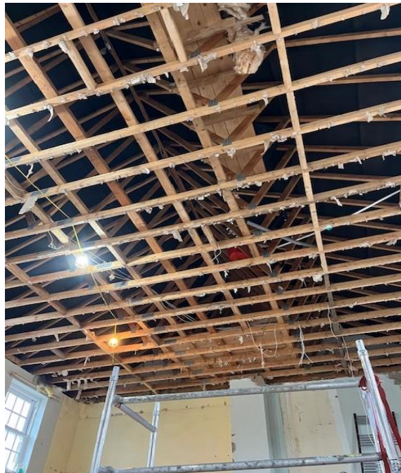
Removal of ceiling of roof void in main house
