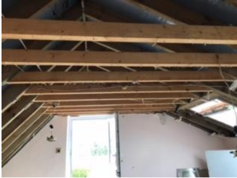
And in garage attic space
