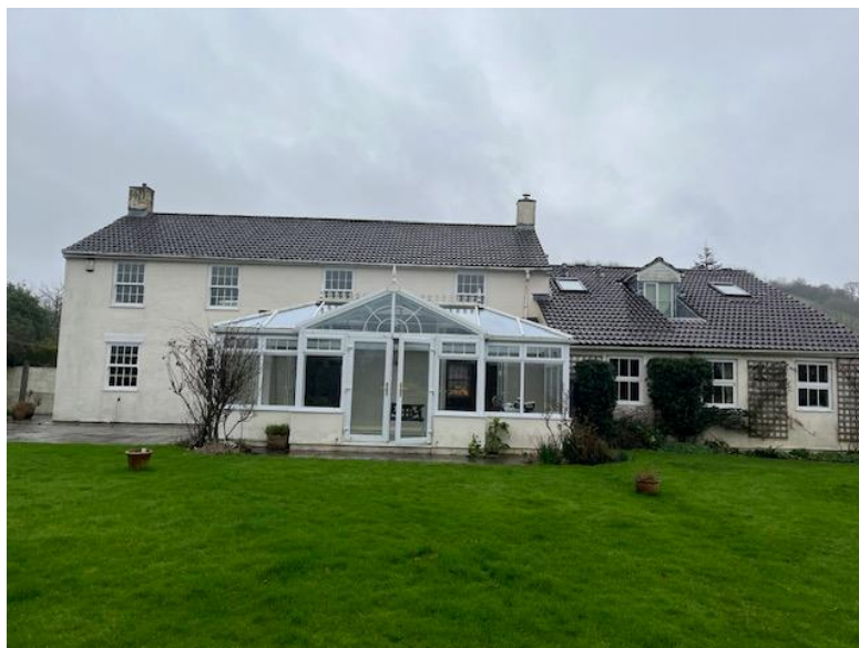
Conservatory and building to the right to be demolished and replaced with new building.
