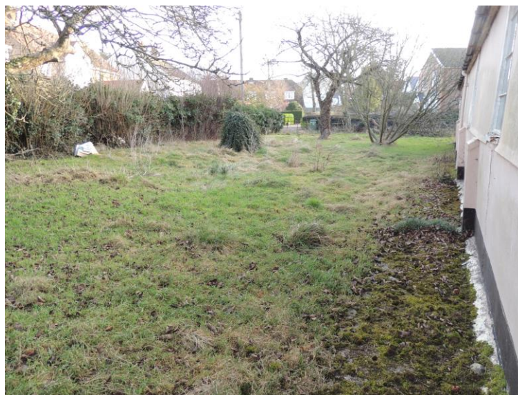
Photo 8: Looking eastwards along northern side of the building
