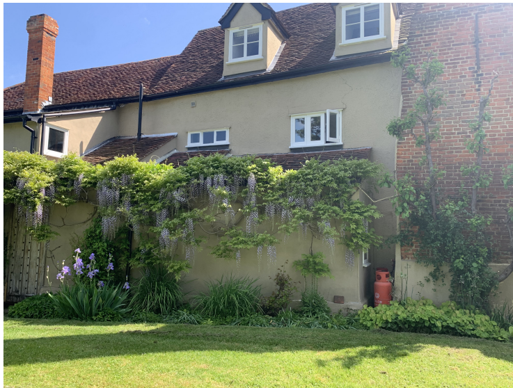
Photo of rear elevation showing modern late single-story addition.
