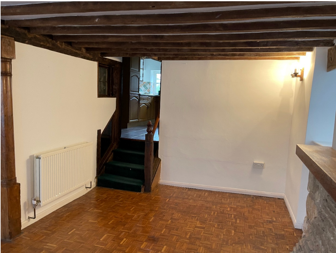
View of existing internal entrance to kitchen
