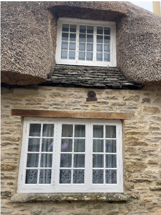
View of front window and dormer
