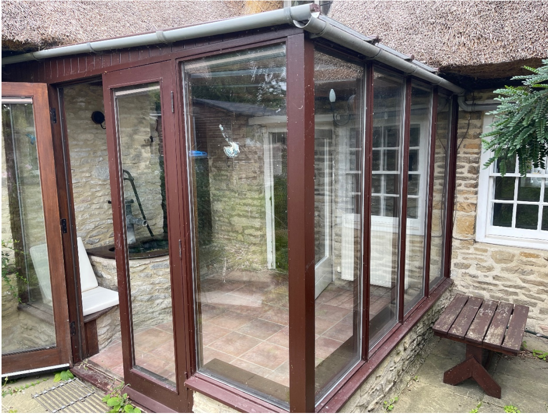
View of existing single storey conservatory
