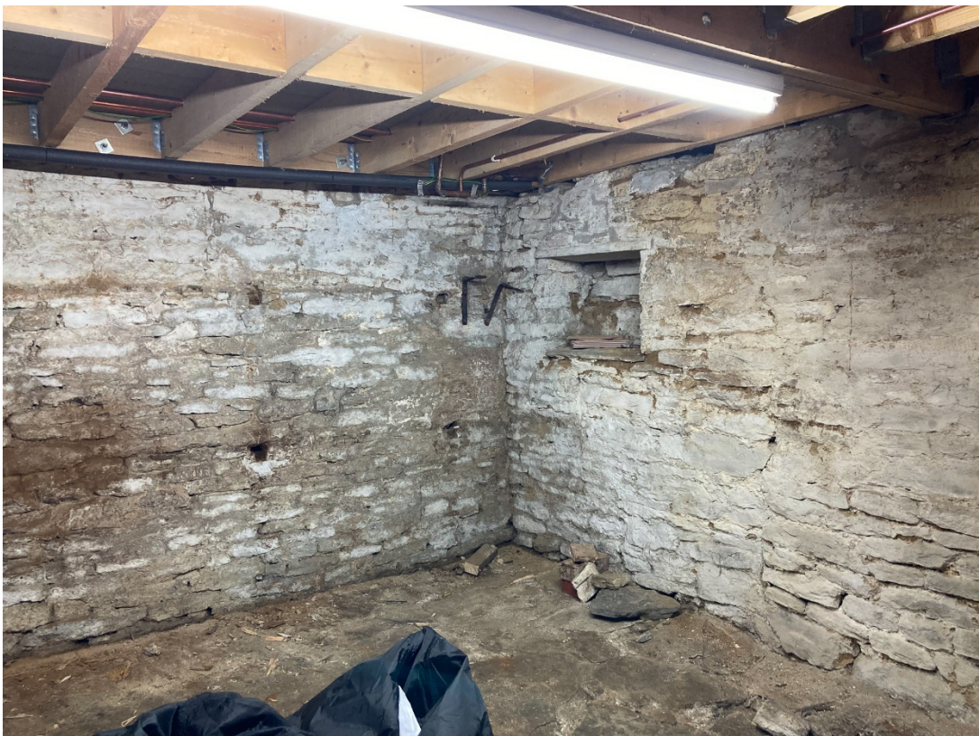
Internal view of existing basement
