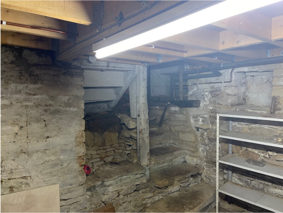
View of existing staircases in basement
