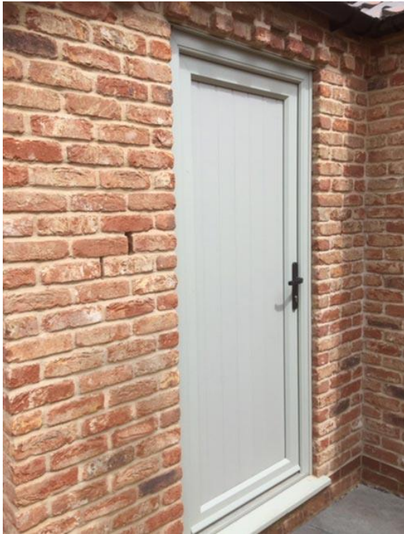
Solid Yeldham door (in white) replacement to the garage
