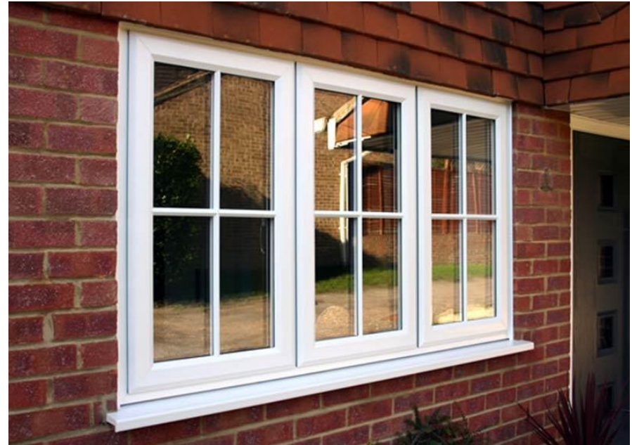
The garage window is to be replaced with a similar style to the original, being a rebated sash in white to match with the proposed door
