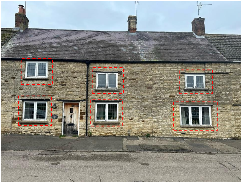
Dashed lines show location of existing windows to be replaced
