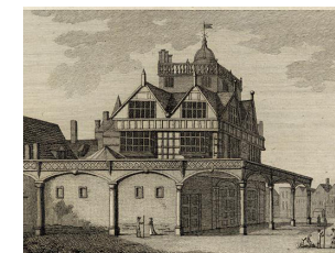
Fig ii: Salisbury Council House
