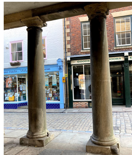
14 Looking East Between columns
