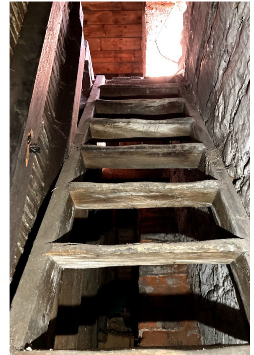
28 Ladder staircase leading to roof void
