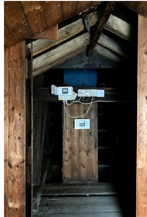
27 Entrance to the clock tower
