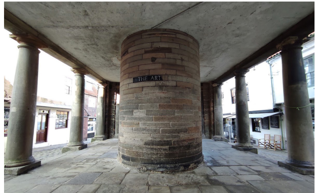
18 Ground Floor: View from Church Street
