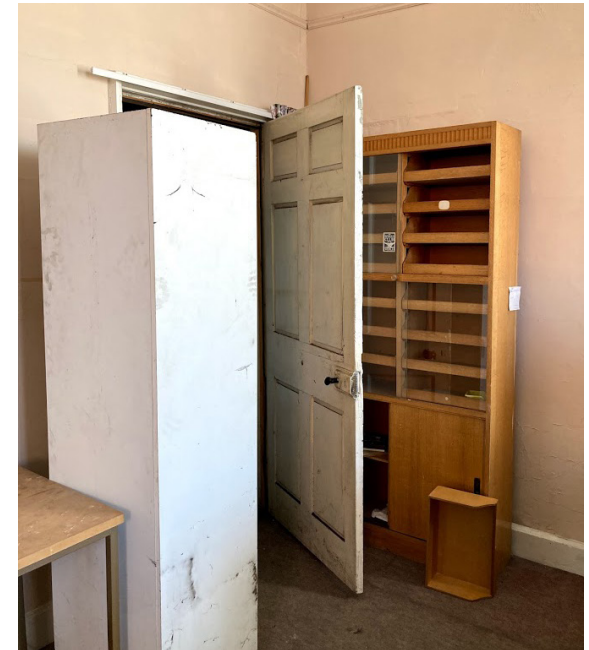
26 Entrance to Roof void/Clock Tower
