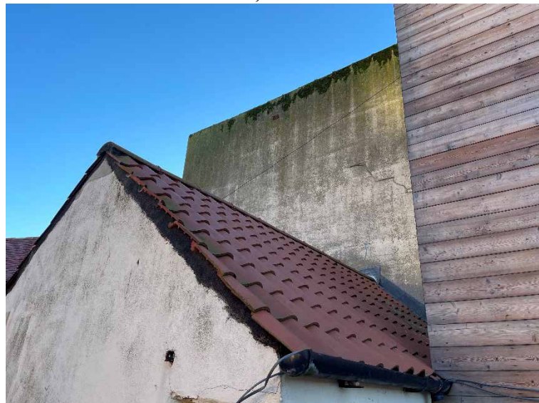
Plate 3 – 39 Sandside, north and west elevation
