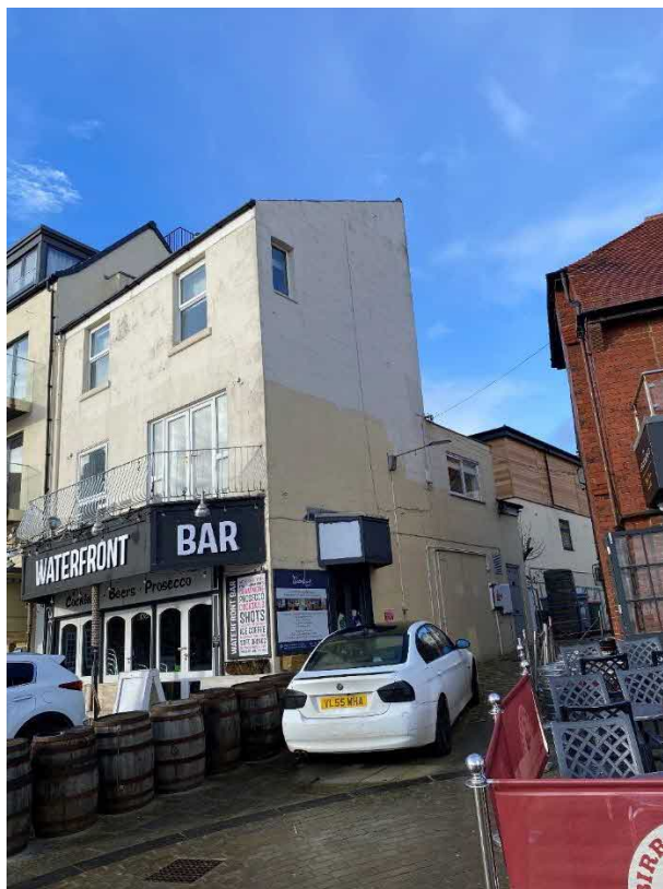
South East Corner
