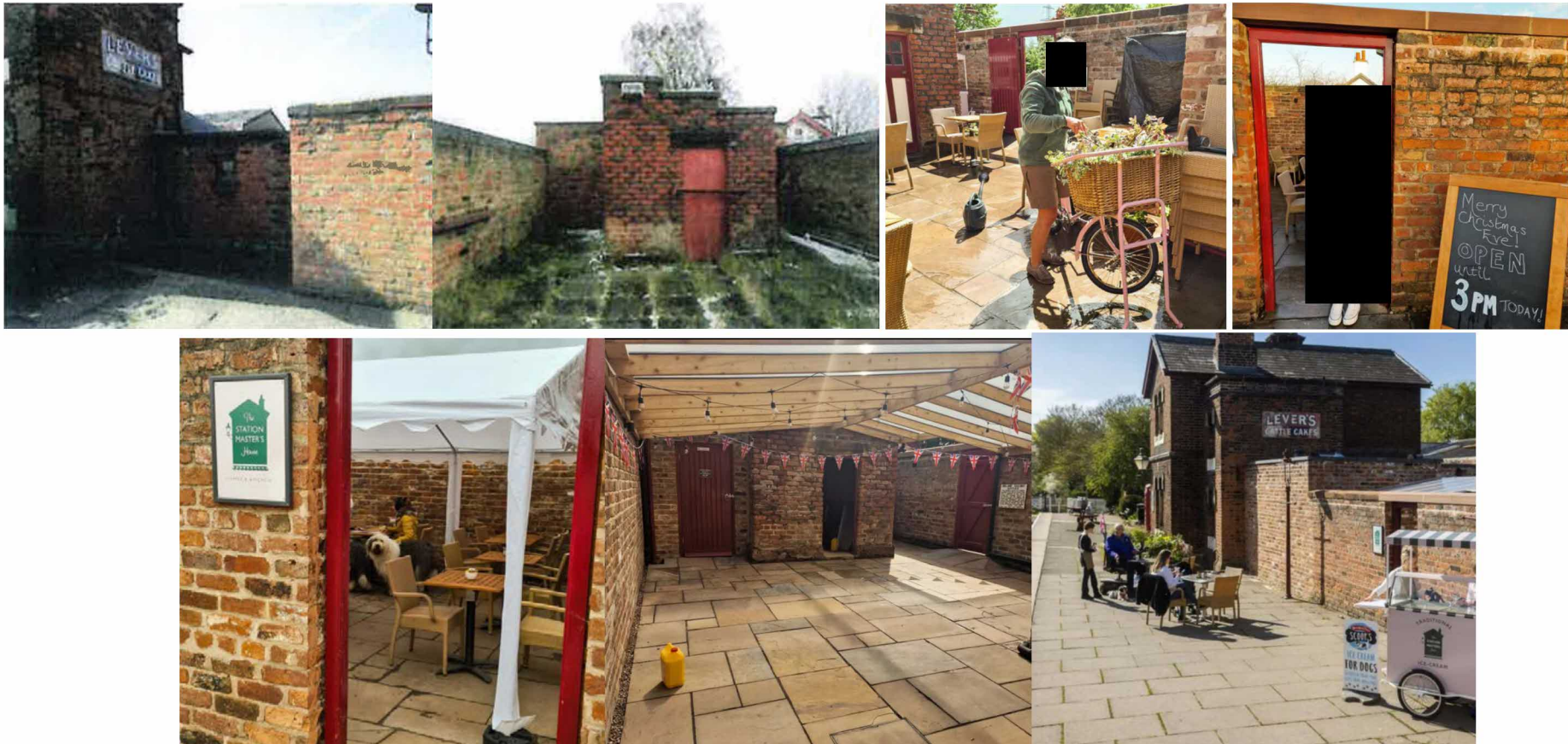
Fig 7. Top from left to right: The first two photographs show the yard prior to the arrival of the Station Master's house. Top right: The Station Master's House courtyard prior to its covering. Without the covering, it can only be used inclemently because of weather.
