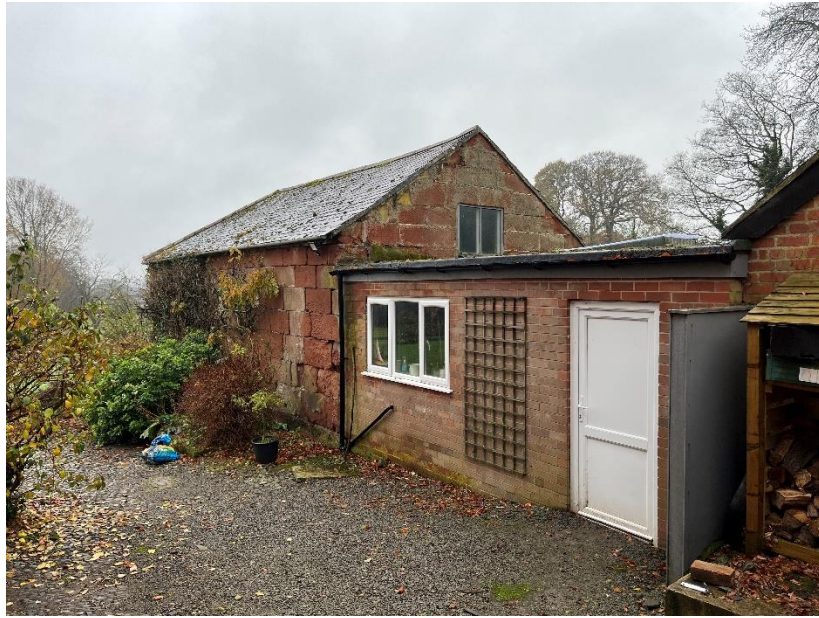
View from the front west end of the Dower House looking south along the east elevation.
