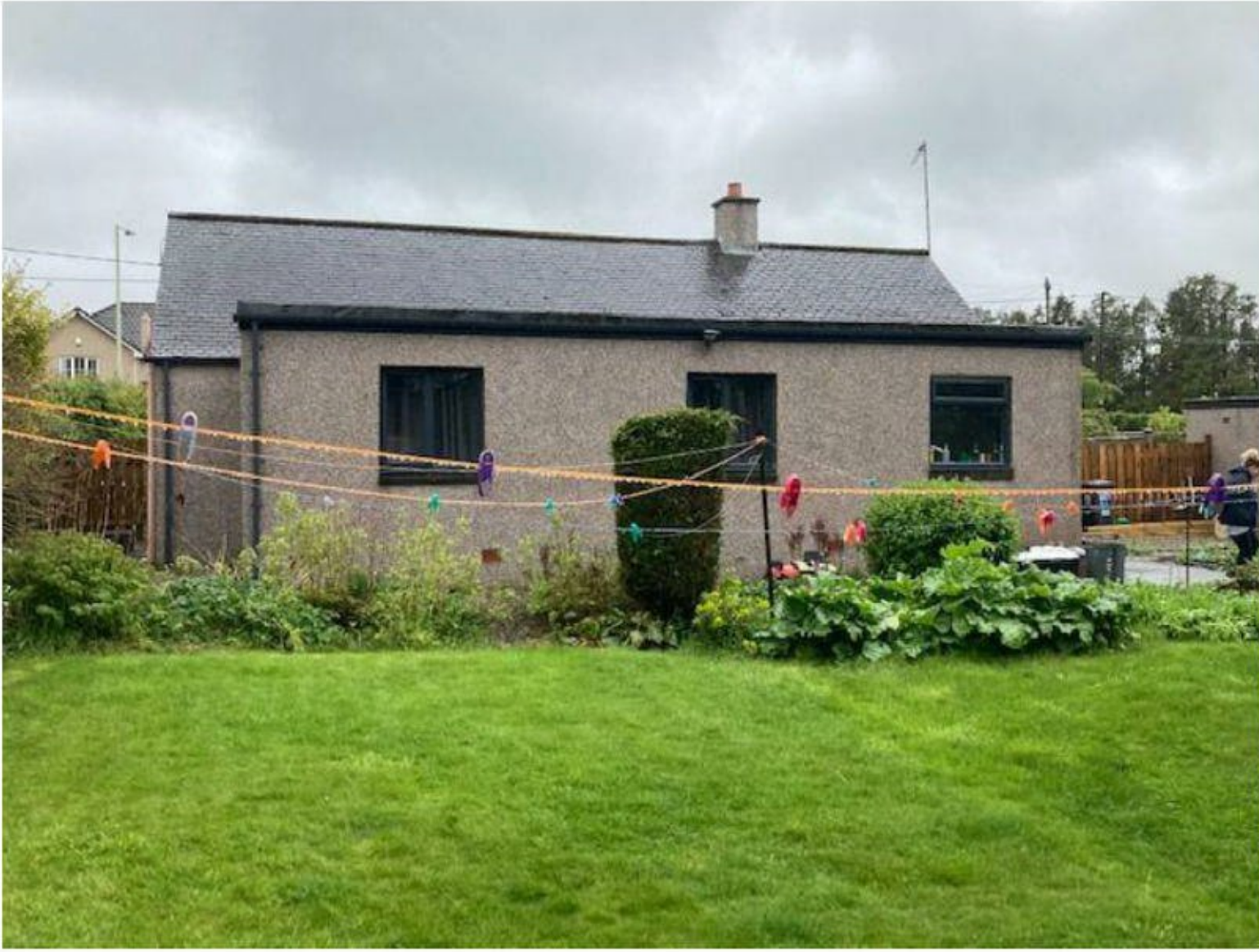
Fig. 8 – North elevation of the house.
