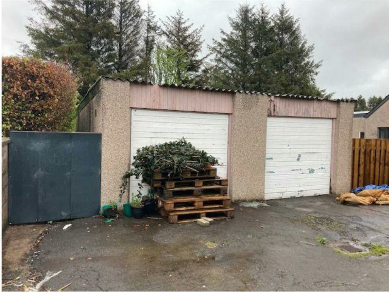
Fig. 10 – South elevation of the double garage.
