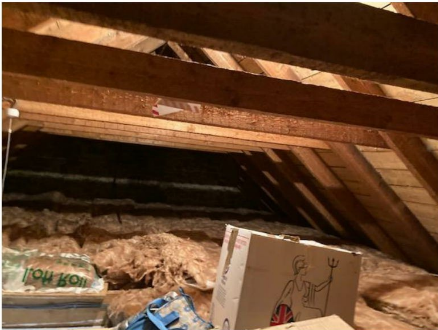
Fig. 13 – Attic space within the house.
