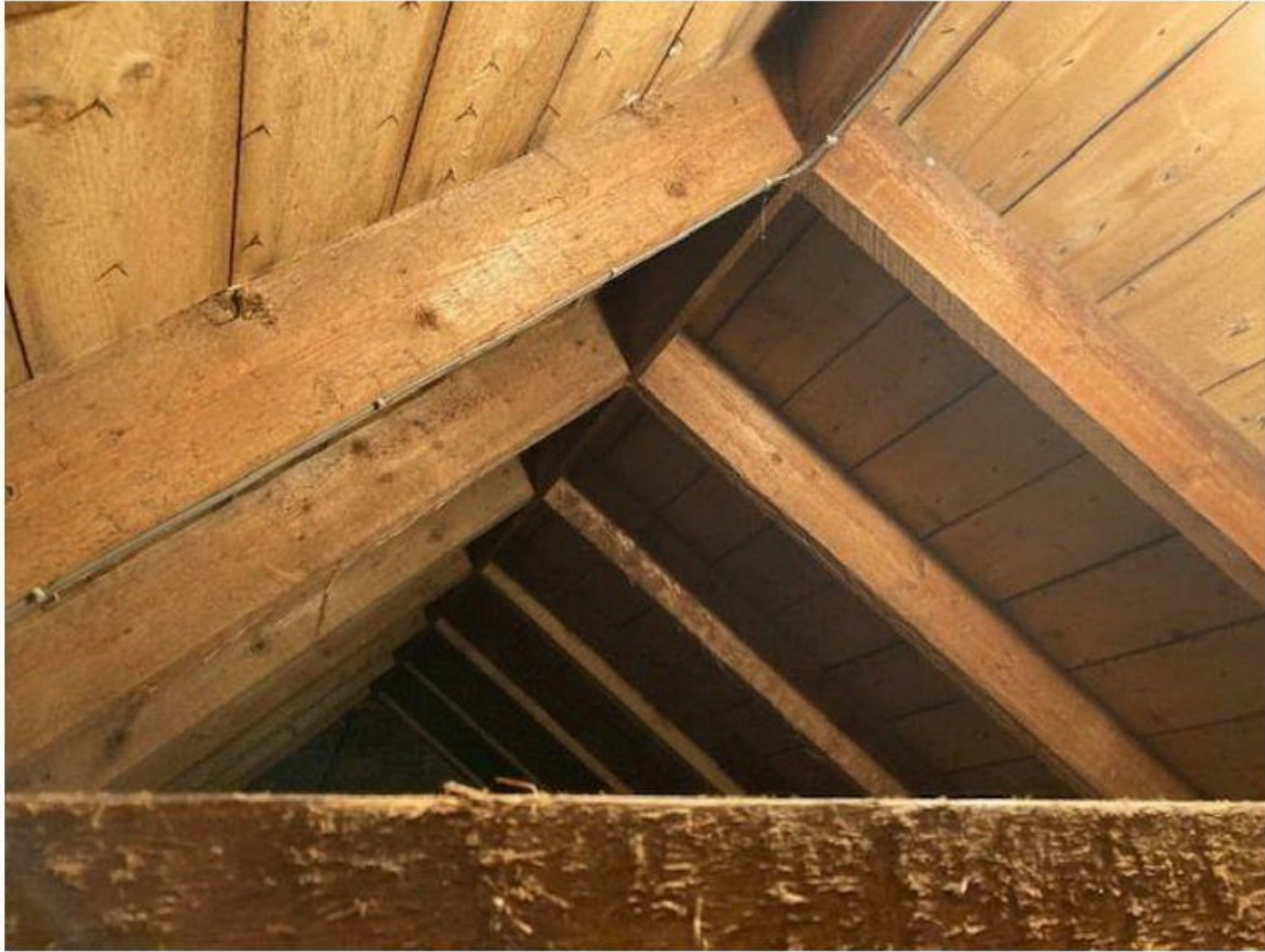
Fig. 12 – Attic space within the house.
