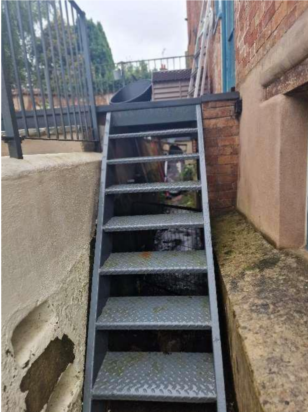
Photo 1 – metal stairs at rear of 2 Corn Mill.
