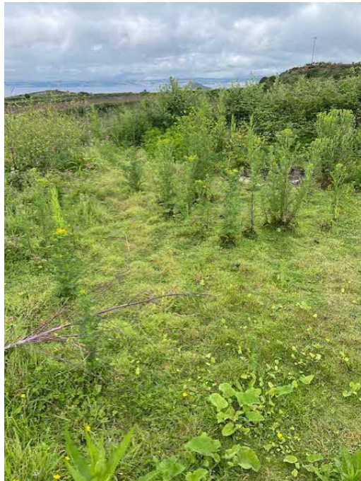
PHOTOGRAPH 4: Uneven ground level and vegetation on site
