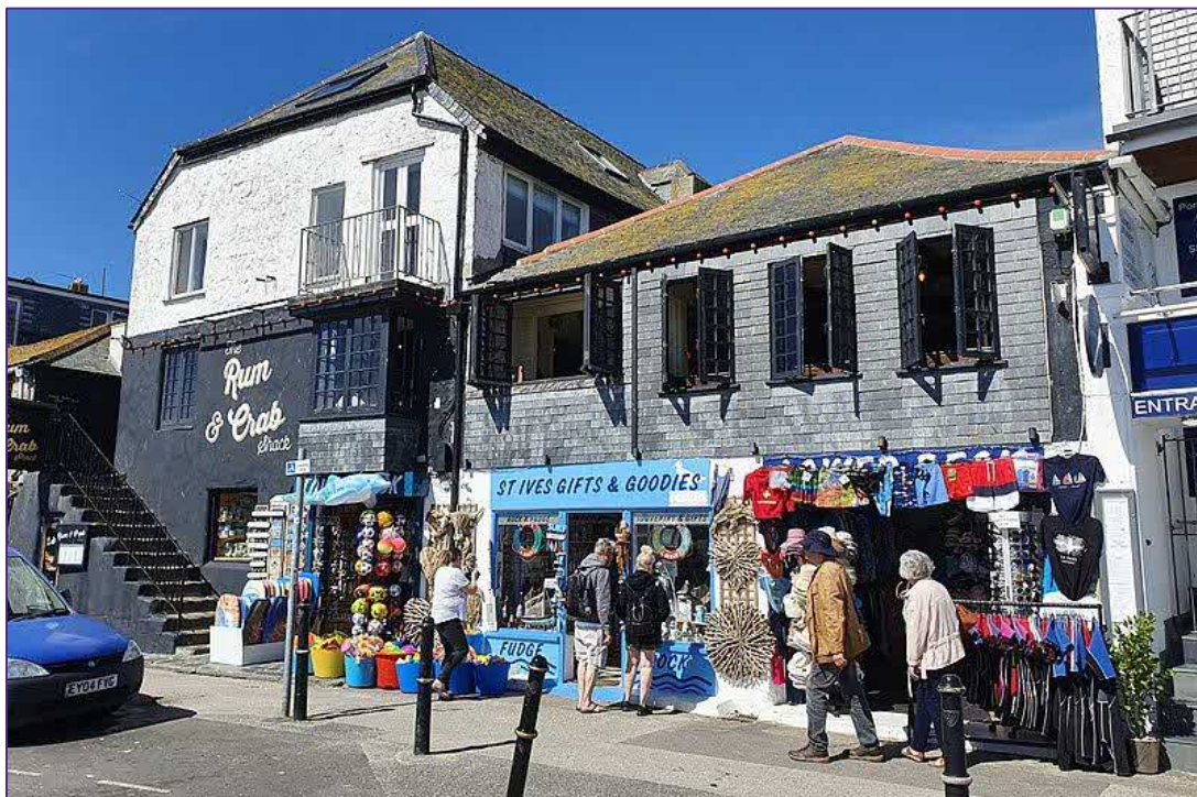
View dating to between May 2018 and June 2022, showing a change to the roof. Some vestiges of the lime slurry coating to the roof slates have survived, but the ridge tiles to the hip appear to be a modern introduction.
