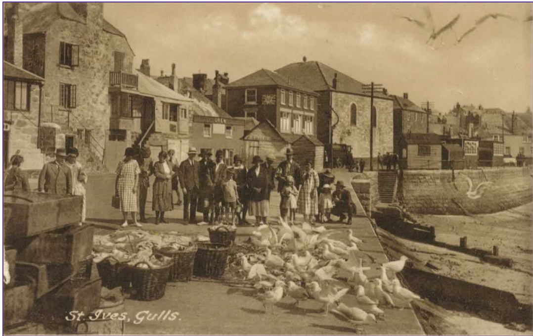
Undated 1930s image, with the Site centre left, showing former external stone steps to first floor.
