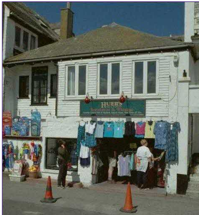
Image dated 8 Jun 2001 (Historic England – Images of England project), showing the Site still pretty much as Listed in 1972, save for the partial infilling of the stone steps to create additional external shop display space. Note slurried and whitewashed slate-hung upper storey and slurried slate roof. According to the subsequent application (01/P/1254 and 01/H/0145 of 2001), the white casements were of PVCu.
