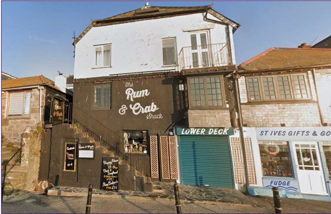
The adjacent Rum & Crab Shack and Lower Deck (Listed as The Copper Kettle and Wimpey Bar) today, with external stone steps visually prominent.
