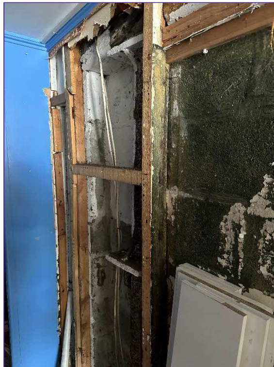
Detail of the concrete-block spine wall.
