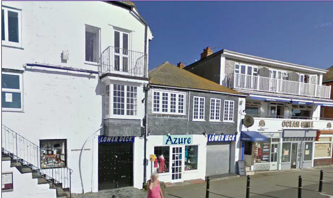
Image showing the Site in June 2009. By this time the balcony opening had been filled in with new bi-fold windows and the shopfronts had been amended. The only historic fabric remaining visible at this time is the slurried slate roof.
