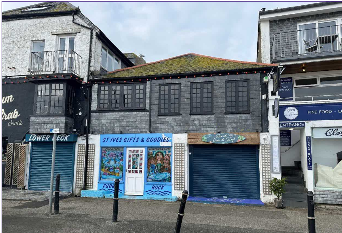
View of the Site (Listed as Premises occupied by Mayfields and Bookshop) today.
