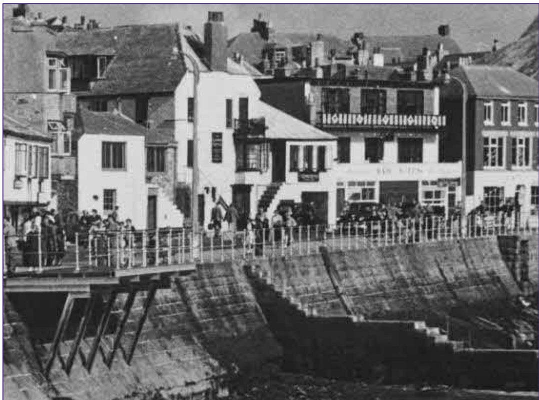
Image dated 1953, with the Site to centre, clearly showing the external stone steps and new first-floor fenestration.
