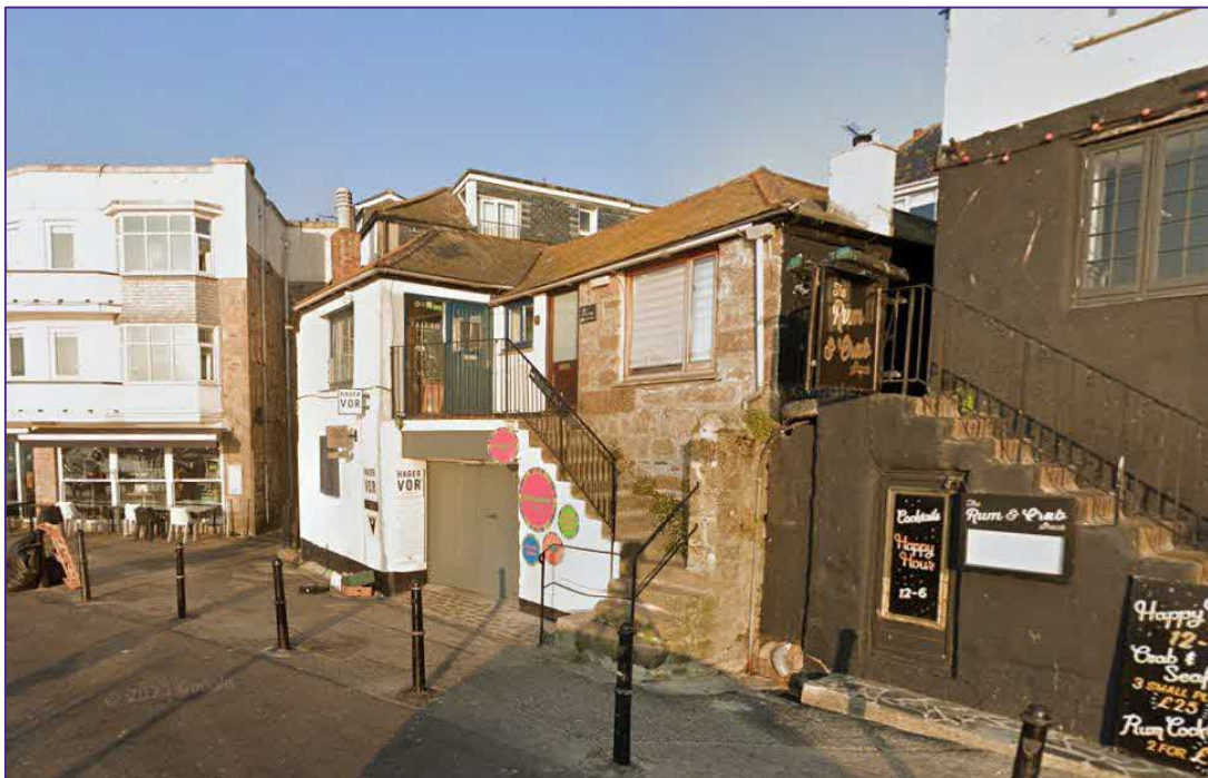
Hager Vor and 2 Rose Lodge (Listed as Rose Lodge Studio) today, with external stone steps prominent.
