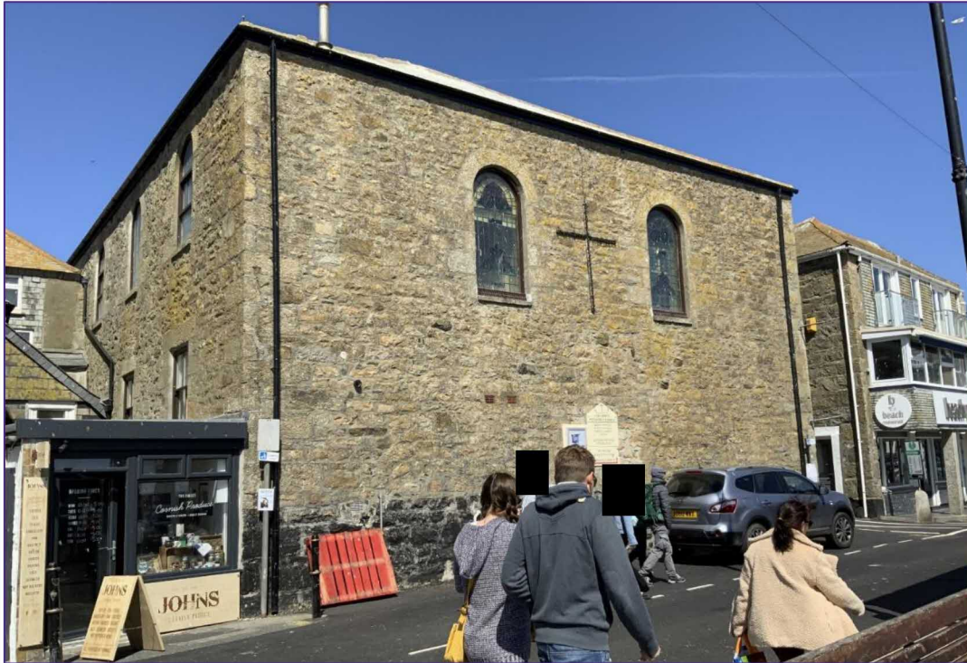
The rear of the Fore Street Methodist Church (Listed as The Primitive Methodist Church, no.1 Fore Street ) facing onto The Wharf.
