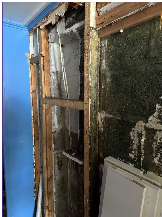
Detail of the concrete-block spine wall.
