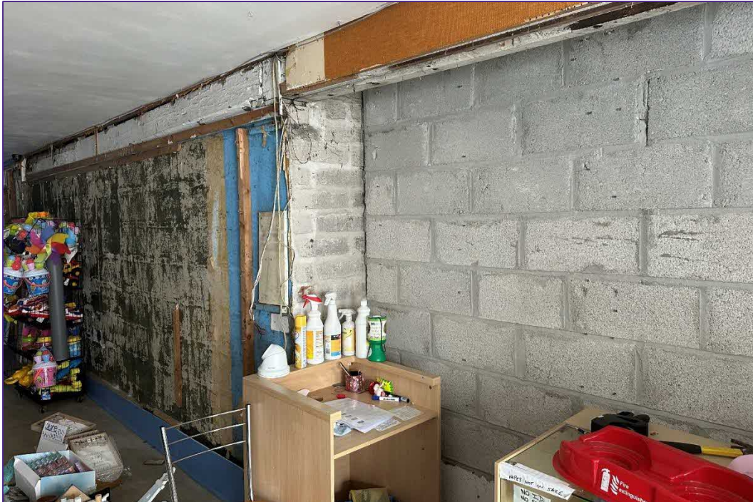
View of the concrete-block spine wall between the units.
