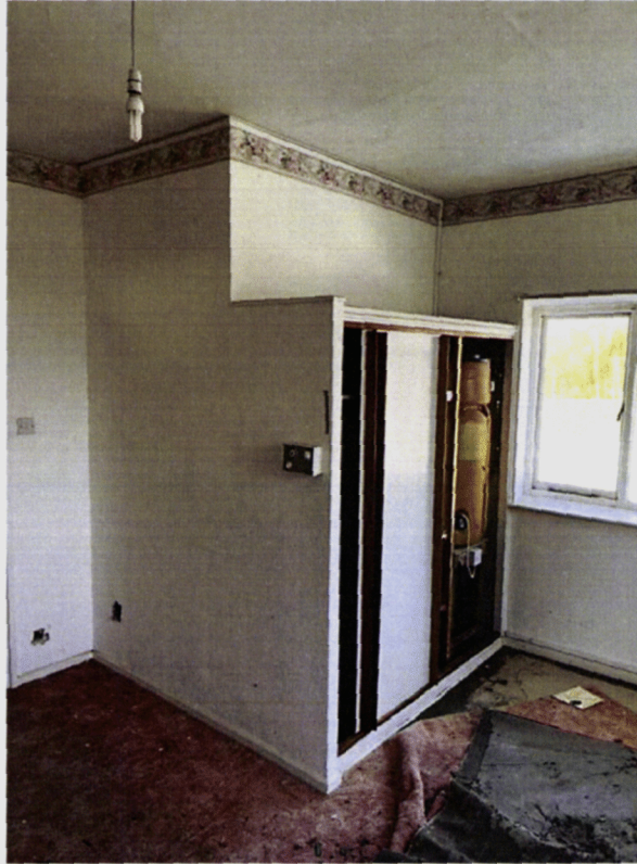
Timber stud partitions surrounding existing bathroom viewed from bedroom 1
