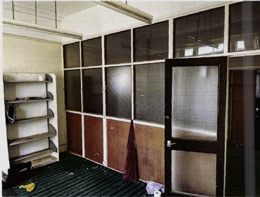
Partition between office 1 and 2 is non loadbearing
