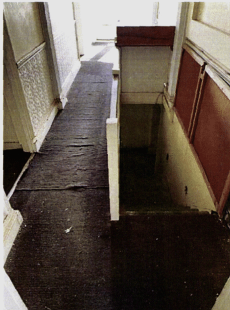
Existing stair opening to be infilled to create ground floor space
