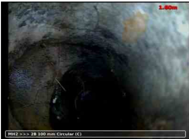
3, 00:00:31, 1.60 m Junction at 9 o'clock, diameter: 100mm, Junction to SWG
