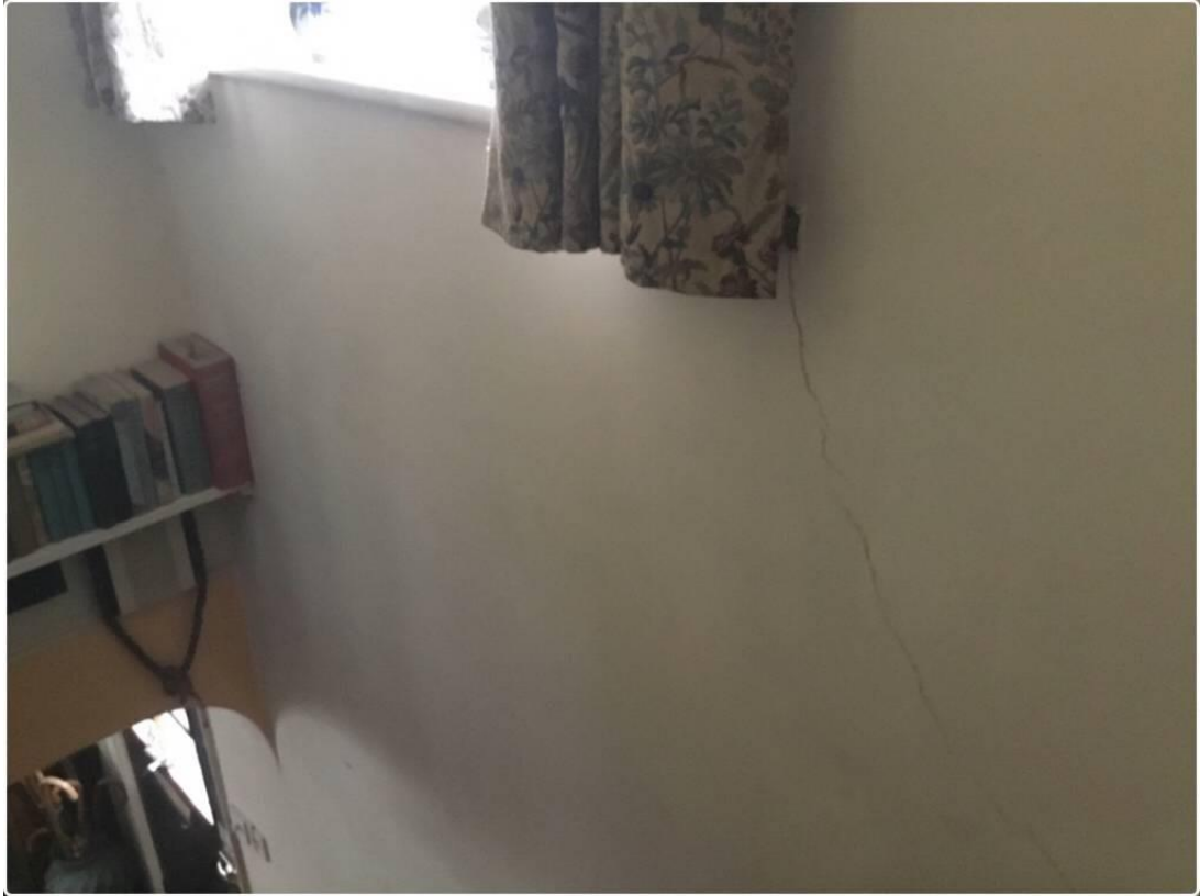
Stair well to left hand side
