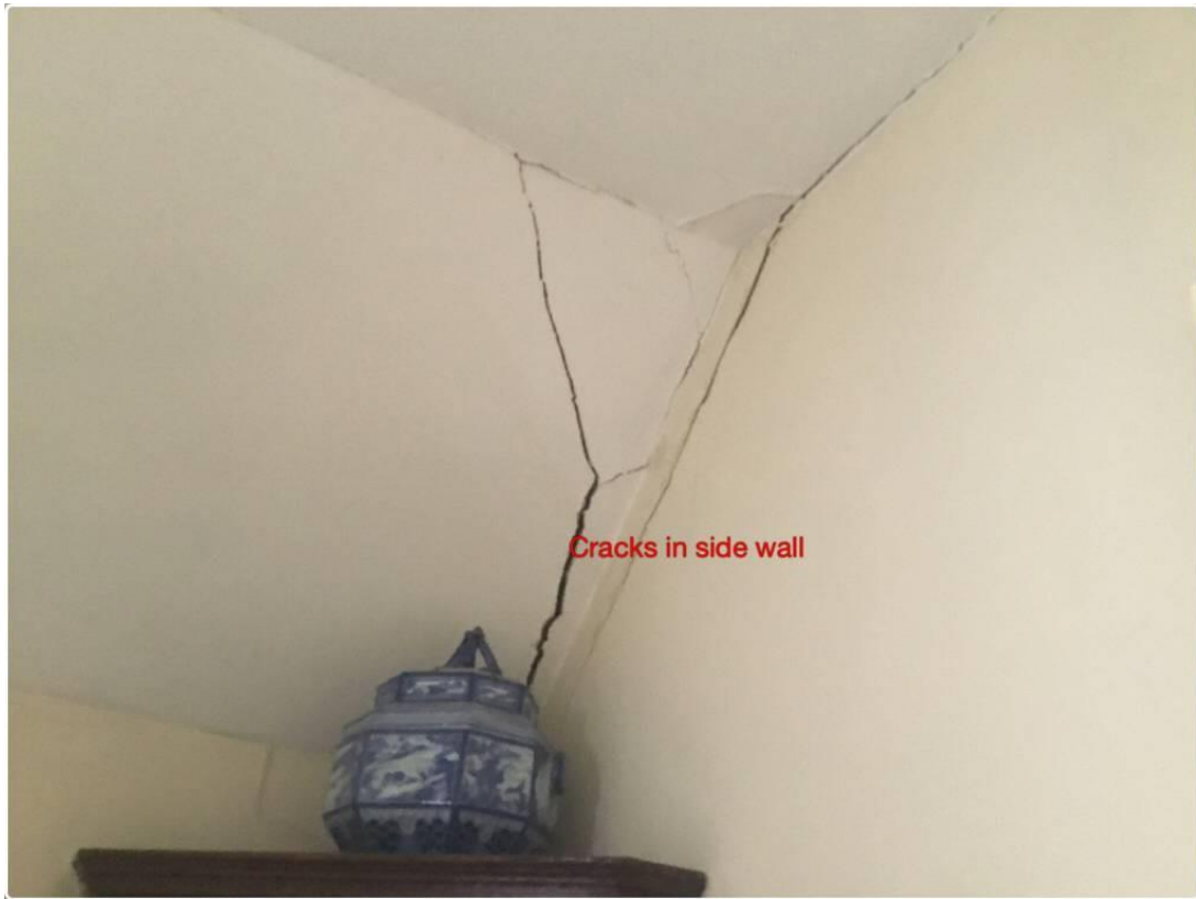
Landing at head of stairs
