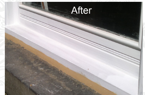
New bespoke timber spliced in with primer coat ready for painting
