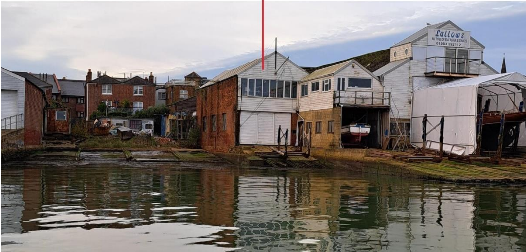
Waterfront view – showing boatshed to be demolished
