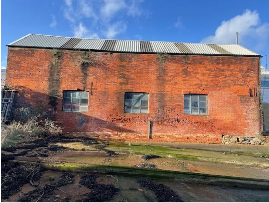
Boat shed 2 to be demolished
