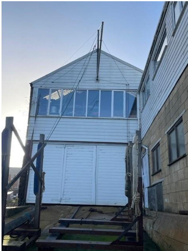
Modern white-painted timber cladding on waterfront elevation of boatshed 2
