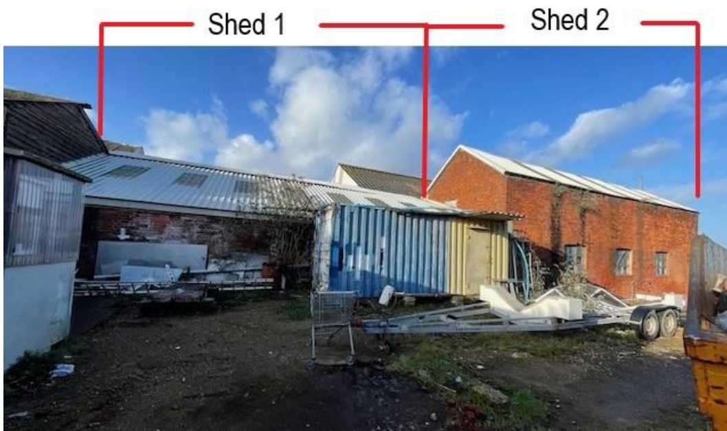
Sheds 1 & 2 to be demolished
