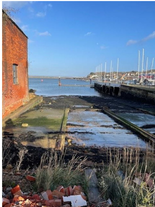
Existing disused maintenance slip – works scheduled for Stage 3
