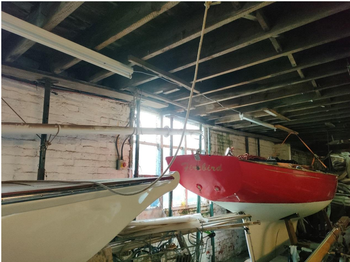
Image 9 Ground floor, propped floor joists.
