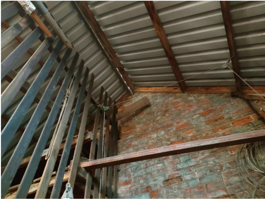
Image 3 Upper floor, view on gable wall.
