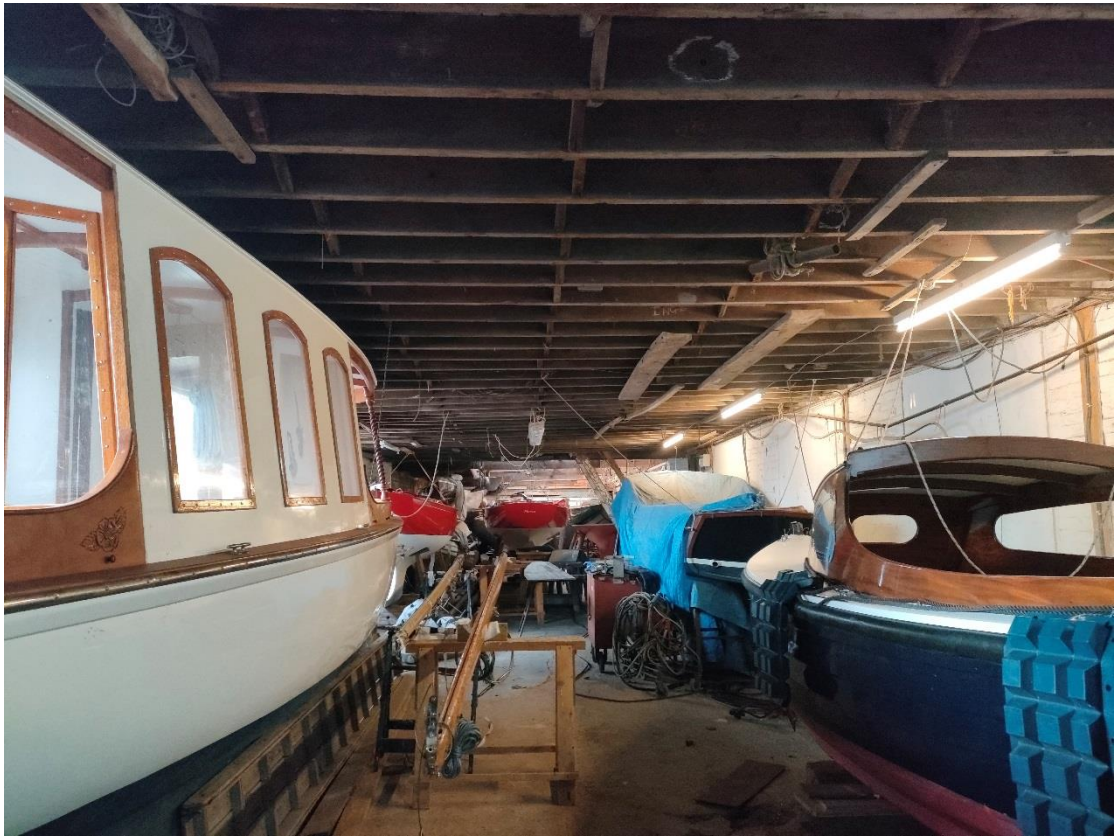
Image 8 Ground floor, general view.
