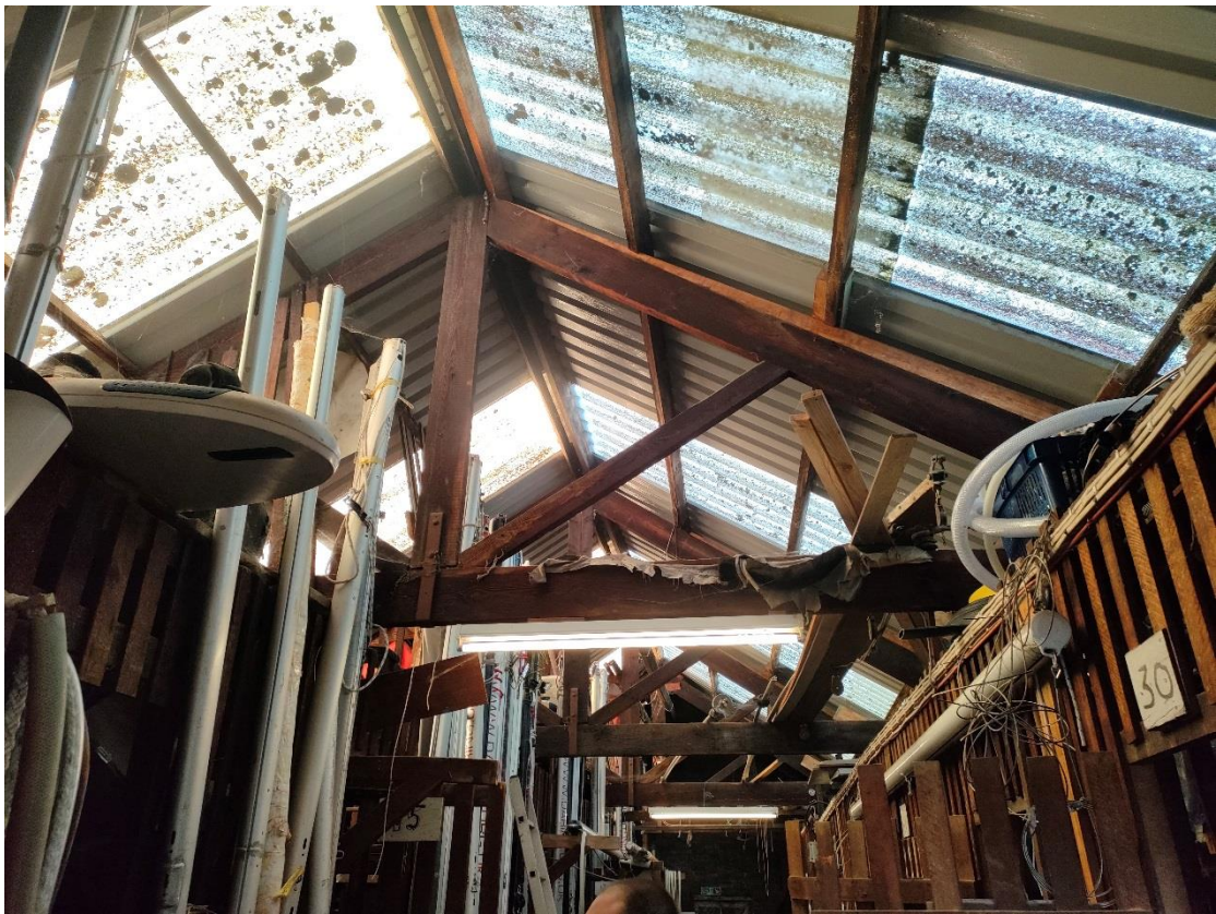
Image 2 Upper floor, view on roof structure.
