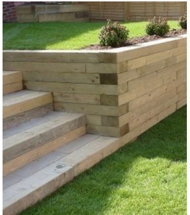
example: sleeper retaining wall rear garden
