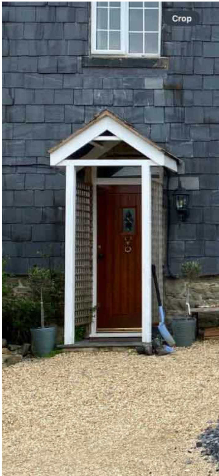
B_Ministers House Side Entrance and Porch
