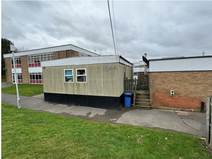
Photo 4 – Existing east and northern facing elevations.
