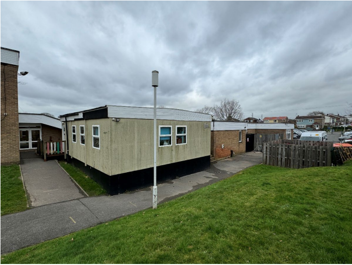
Photo 3 – Existing southern and eastern facing elevations.
