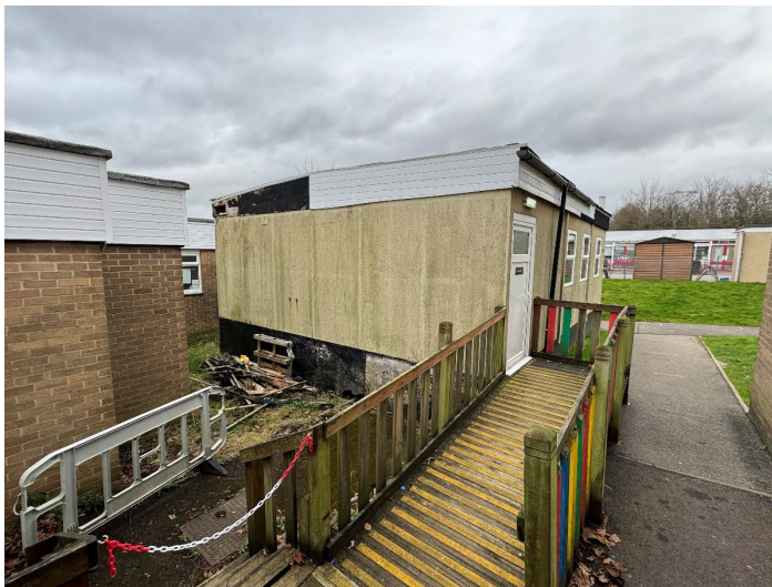
Photo 5 – Existing west and southern facing elevations.
