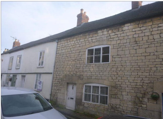
Plate 1: View of the North Elevation of the House
