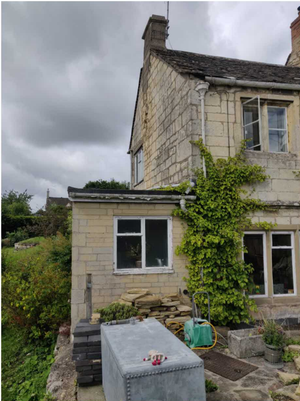
Front elevation of the modern extension.
