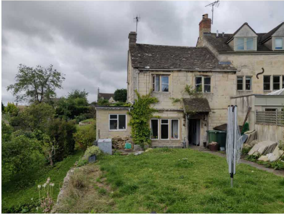
Overall view of Bentley Cottage.
