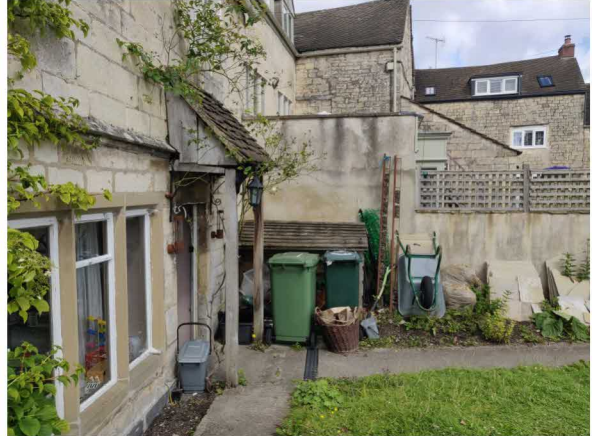
View towards the neighbouring properties.
