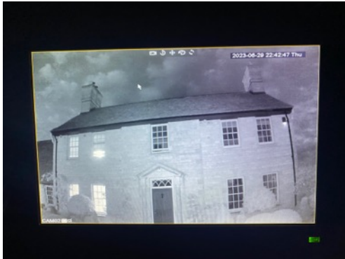
Photo 19: Example infrared camera view – B1
