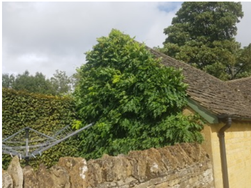
Photo 13: B2 - SW facing gable end
