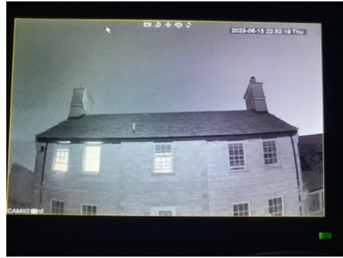
Photo 20: Example infrared camera view – B1
