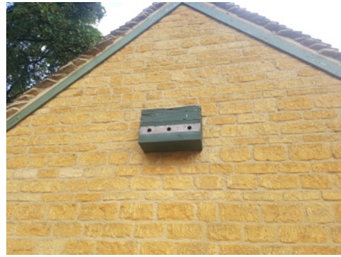
Photo 14: B2 - Sparrow terrace on NW facing gable end wall
