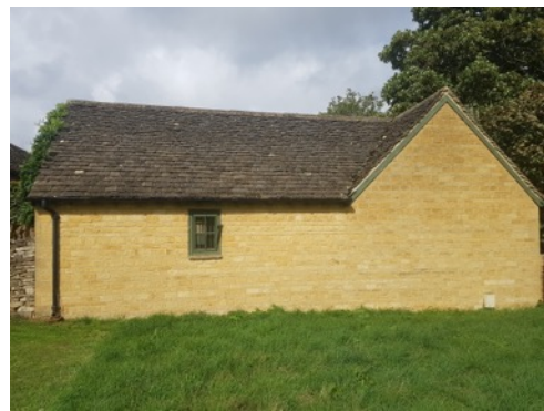
Photo 12: B2 - SE facing elevation
