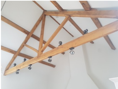
Photo 7: B1 - Vaulted ceiling above kitchen within single storey wing
