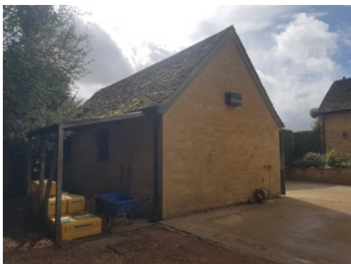
Photo 15: B2 - Viewed from NW
