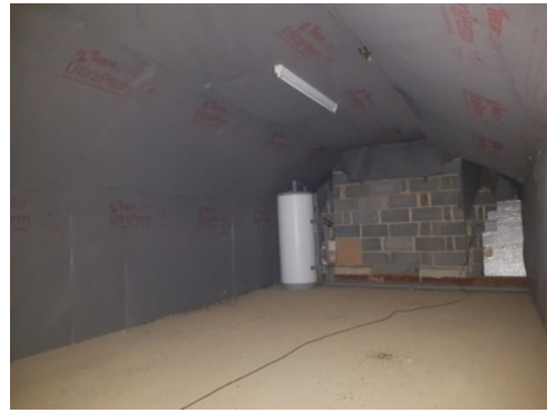
Photo 8: B1 - Loft void
