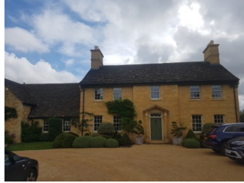
Photo 2: B1 - Front NW facing elevation
