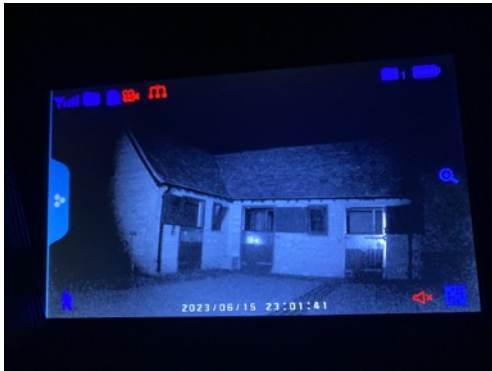
Photo 23: Example infrared camera view – B2
