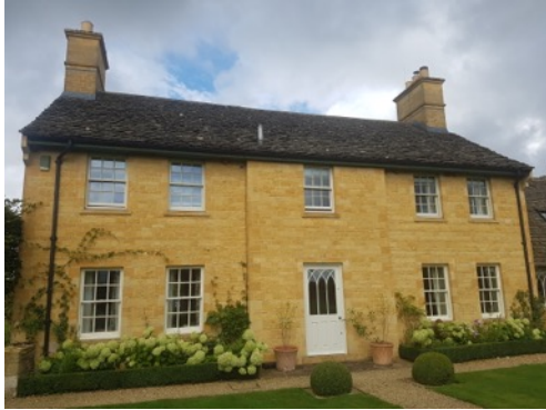
Photo 1: B1 - Rear SE facing elevation of two storey wing.
