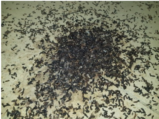
Photo 27: Concentration of bat droppings upon loft floor of B1. July 2023
