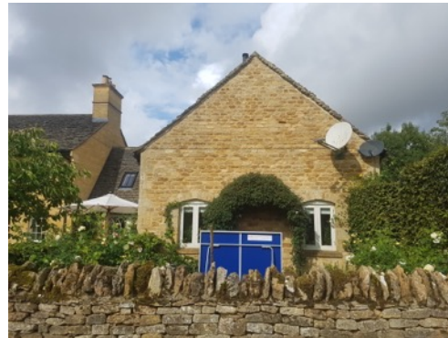
Photo 4: B1 - SE facing gable end wall of single storey wing
