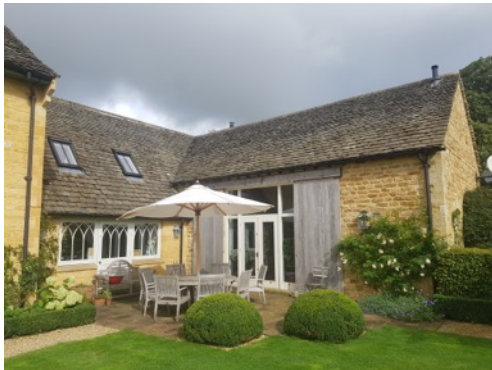
Photo 3: B1 - Rear elevations of single storey wing.
