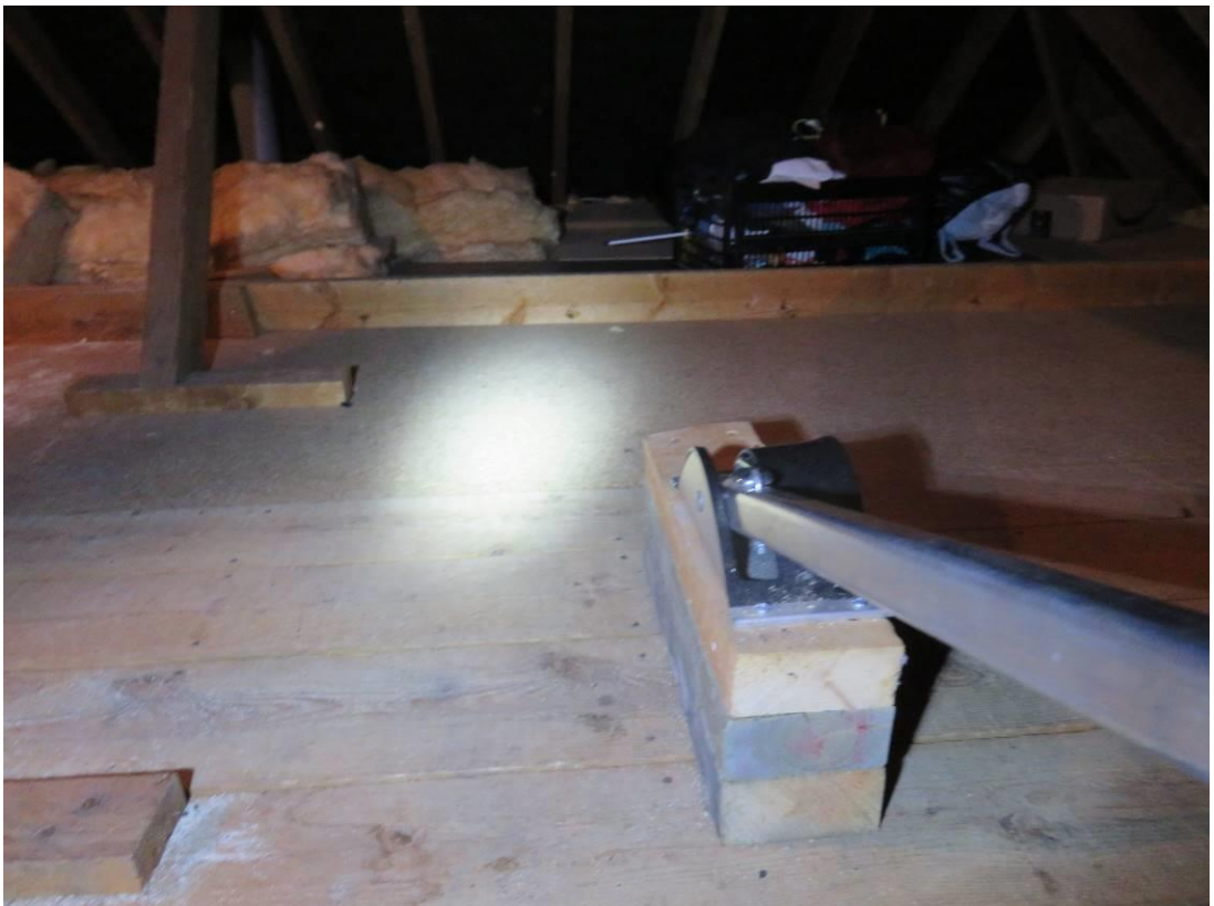
Photo 13/14 internal roof area of building with no long-term accumulation of cobwebs.
