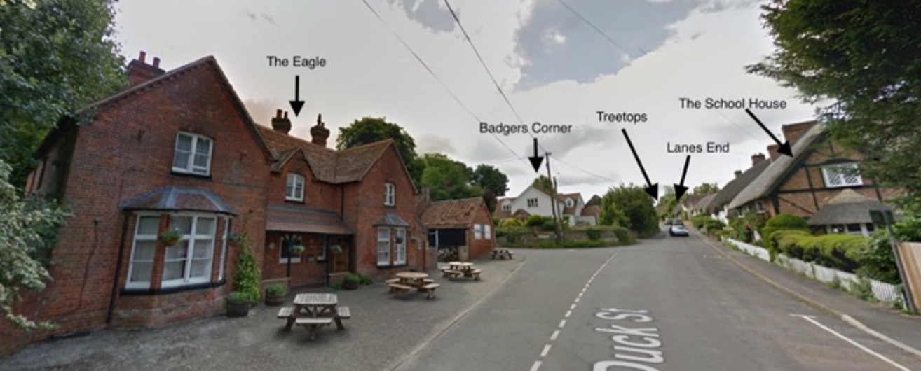
The School House to Lanes End looking south
