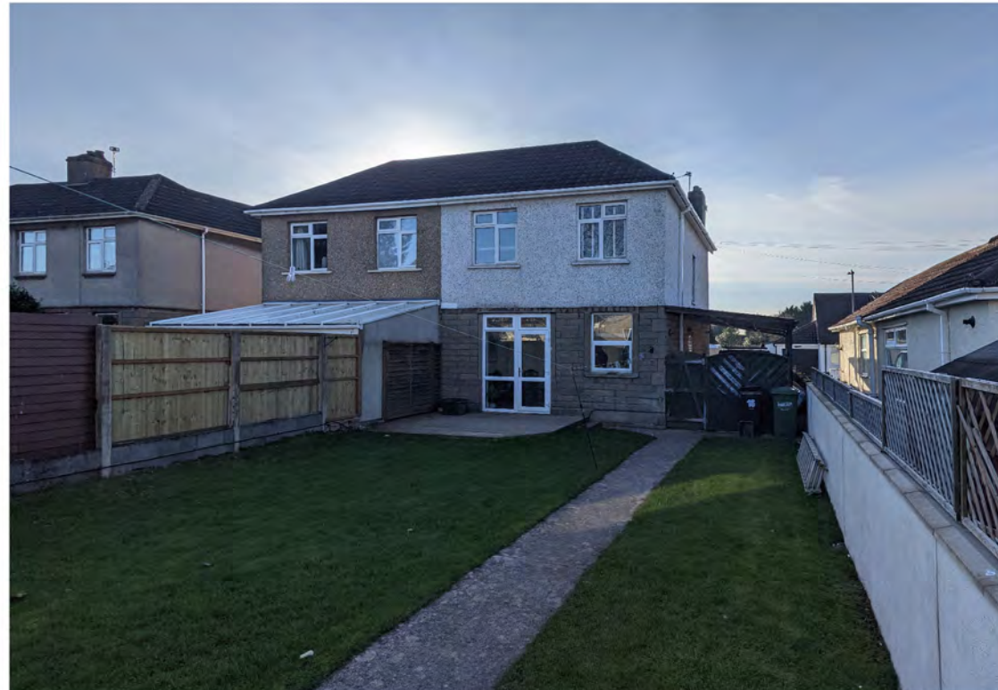
Photo 2 - Rear of House looking from Rear Garden
