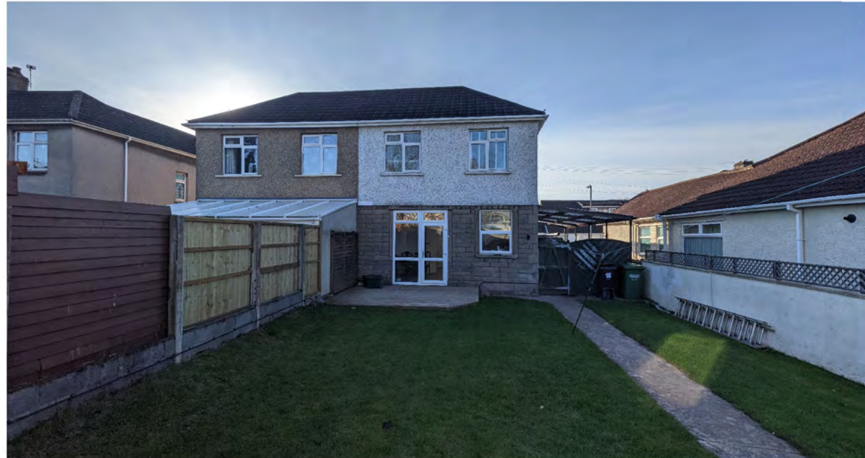
Photo 1 - Rear of House looking from Rear Garden
