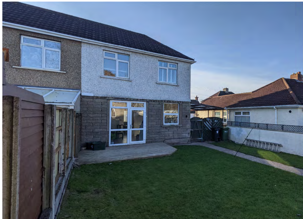
Photo 3 - Rear of House looking from Rear Garden
