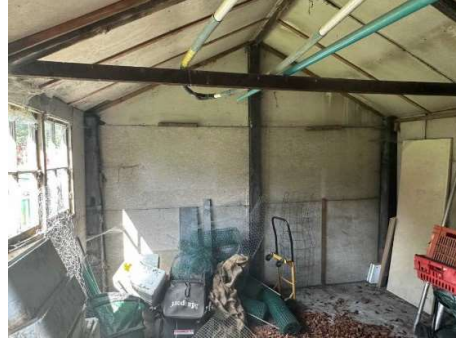
Images: Left – Corrugated Steel Workshop. Right –Interior of Workshop with asbestos wall and ceiling panelling.
