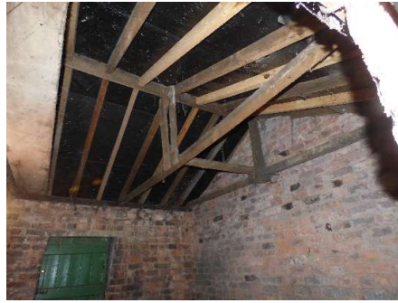
Images: Left – Brick Garage and Coal Shed. Right –Interior of Coal Shed with damaged roof and asbestos ceiling panelling.
