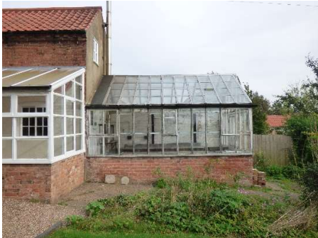
Images: Left – Greenhouse and Stainless-Steel chimney.
