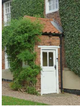
Image: Existing Porch to the front of the property.
