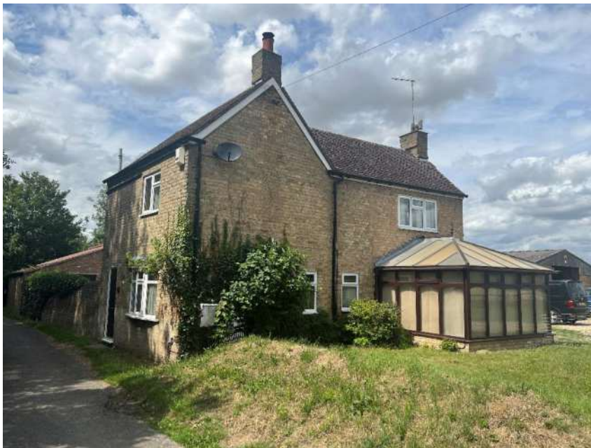
Dwelling – south and east facing facades
