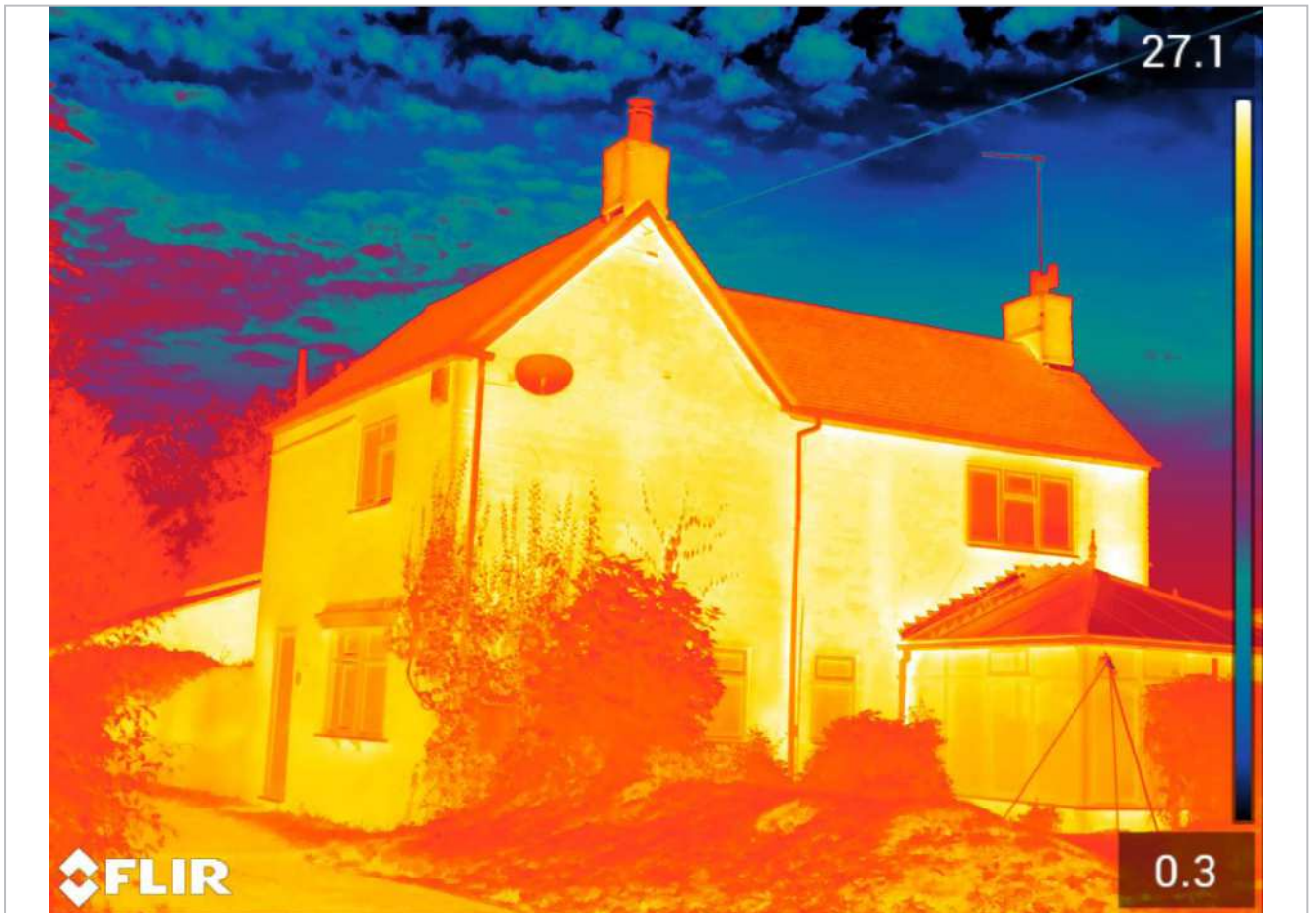
FLIR T1020 (1024 x 768 pixel resolution) with 45 degree lens = bat in flight detection distance of 104 m. Camera located 24 m from furthest point of building
