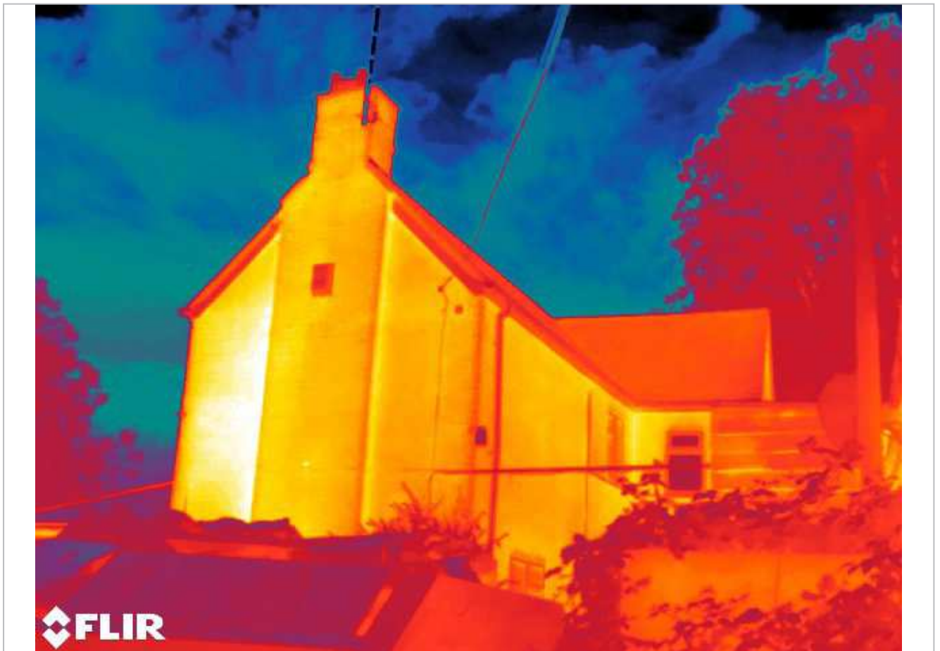
FLIR T860 (640 x 480 pixel resolution) with 42 degree lens = bat in flight detection distance of 66 m. Camera located 21 m from furthest point of building
