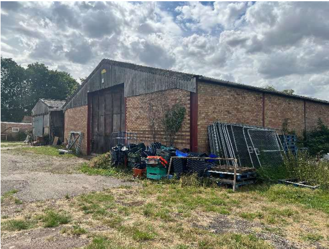
Exterior of the barn
