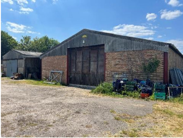
Existing agricultural barns and hardstanding
