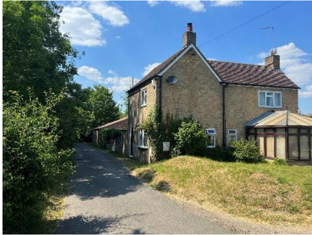
Existing house viewed from Clay Close Lane looking west
