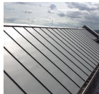
Metal Roof- Zinc
