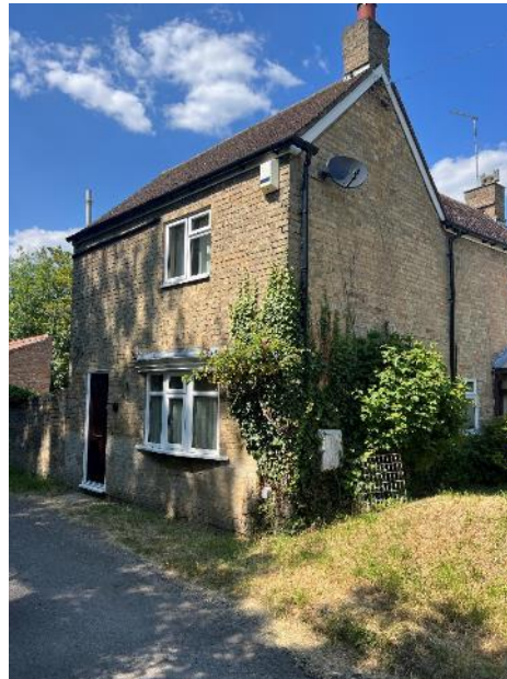
Existing front elevation of house
