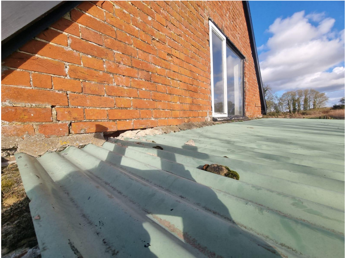
Photo 3: External view of where garage roof is keyed into the gable wall
