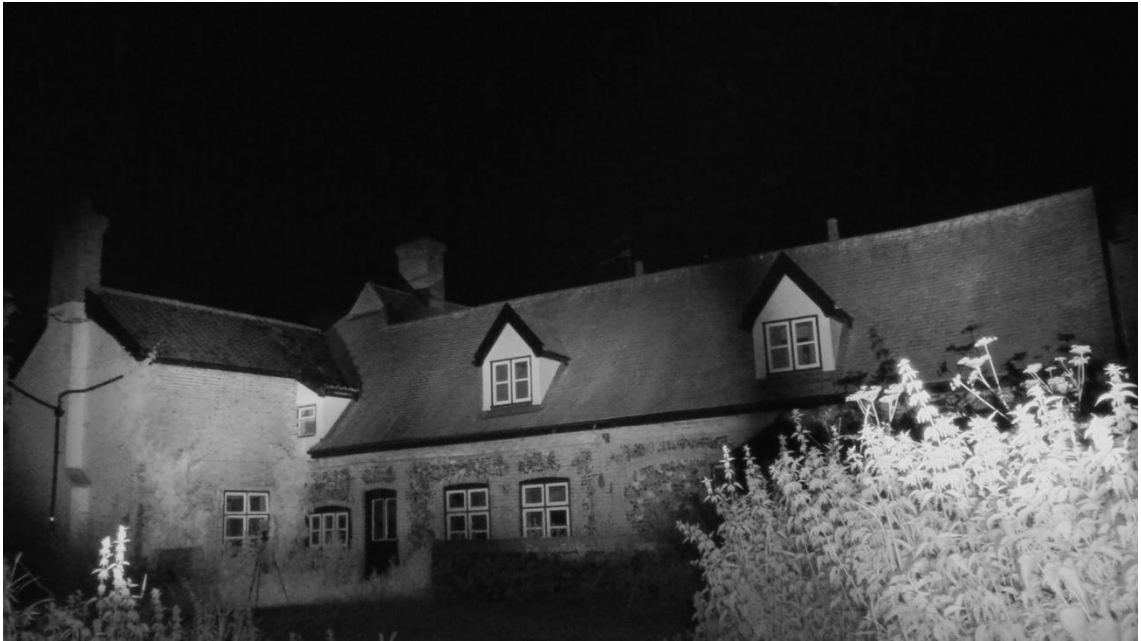
Photo 10 , screenshot from infrared camera on southwest corner. 22 nd June 2023.
